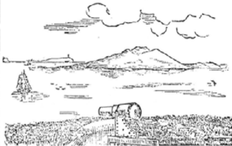
CHALLENHAM BEACH BATTERY.
