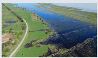
Figure 23. Aerial image of Wairio Wetlands showing high water levels being retained behind the bund wall. The area of open water (top right) is Wairarapa Moana. *Photo: Ducks Unlimited NZ.*
