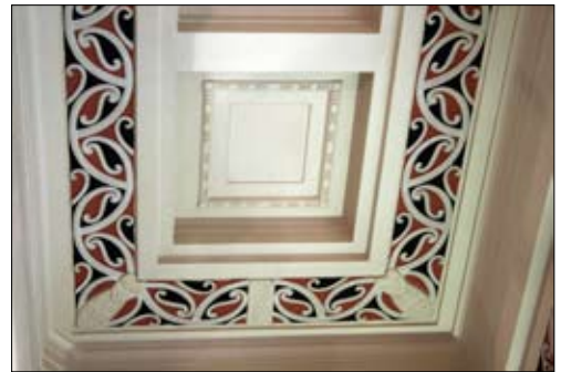
Figure 12. Former Bank of New Zealand Building, detail of ceiling.
