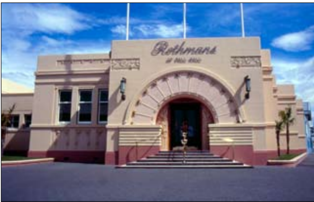
Figure 22. Former Imperial Tobacco Company Building, Ahuriri, built 1933.
