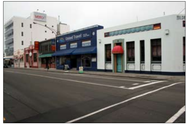
Figure 18. Vero Building on Tennyson with adjacent single-storey buildings dating from 1931 to 1932 on the right.
