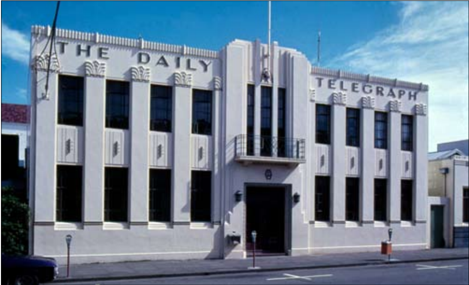
Figure 7. Daily Telegraph Offices, Tennyson Street, built 1932.
