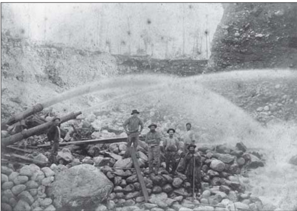
Sluicing on the West Coast, 1880s. Reproduced by permission of the Alexander Turnbull Library, Wellington, N.Z. Ref. no. F-44511-1/2.
