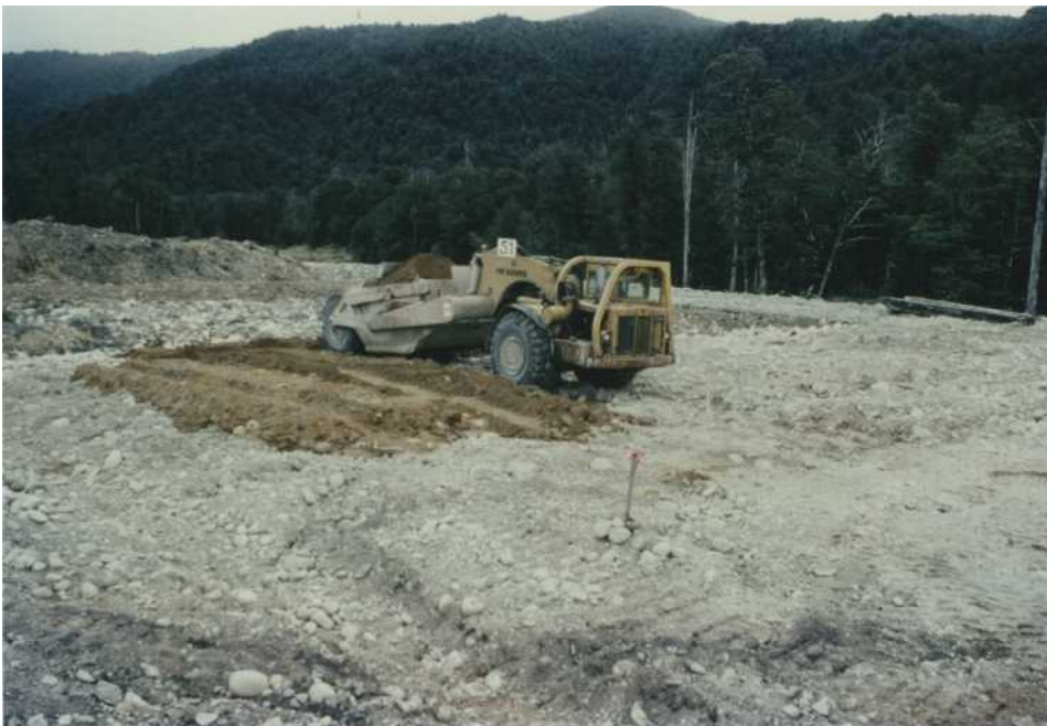
FIGURE 8. SPREADING SUBSOIL OVER COMPACTED SOILS.
