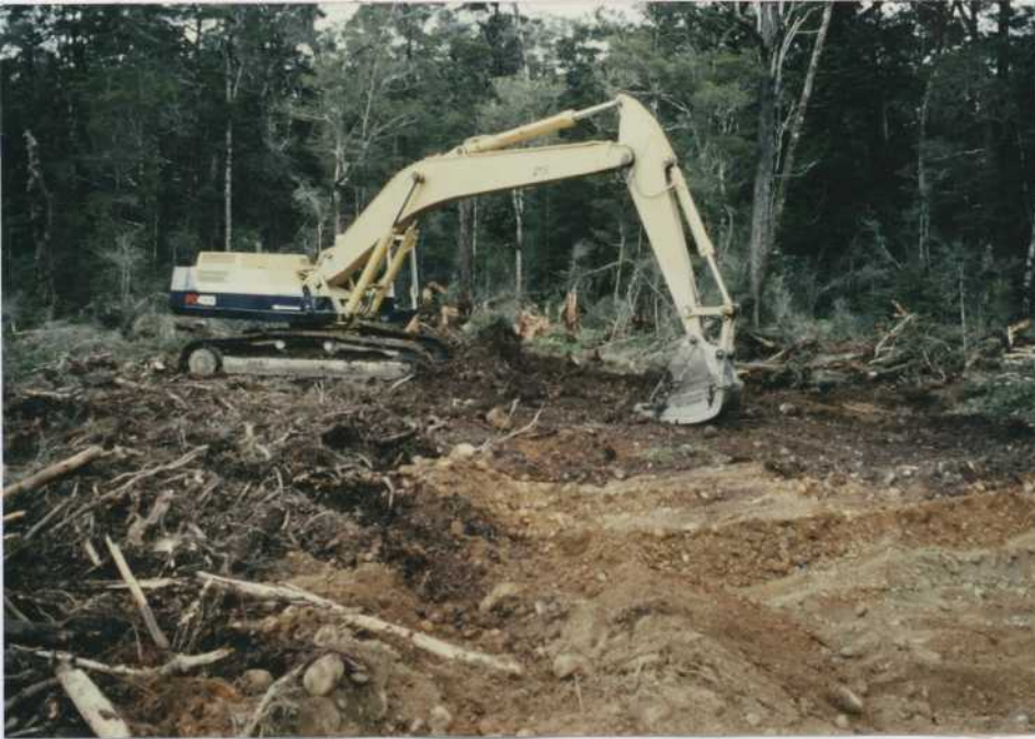
FIGURE 7. STRIPPING SURFACE ORGANIC LAYERS AND TOPSOIL FROM A CLEARED FOREST AREA.
