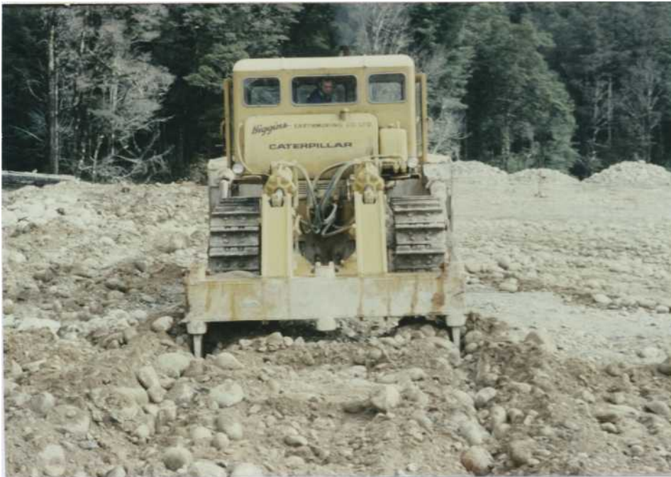
FIGURE 6. RIPPING TO AMELIORATE COMPACTION IN THE GRAVELS.
