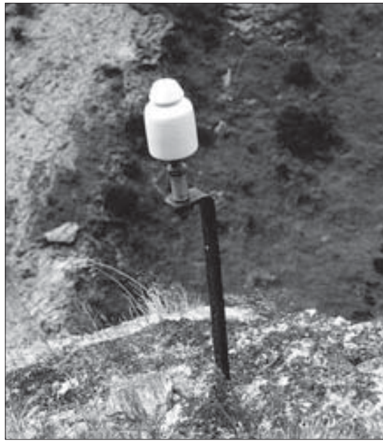
Figure 42. Telephone pole and insulator on the telephone line out to Skippers from Bullendale, 1996. Photo: P. Petchey.
