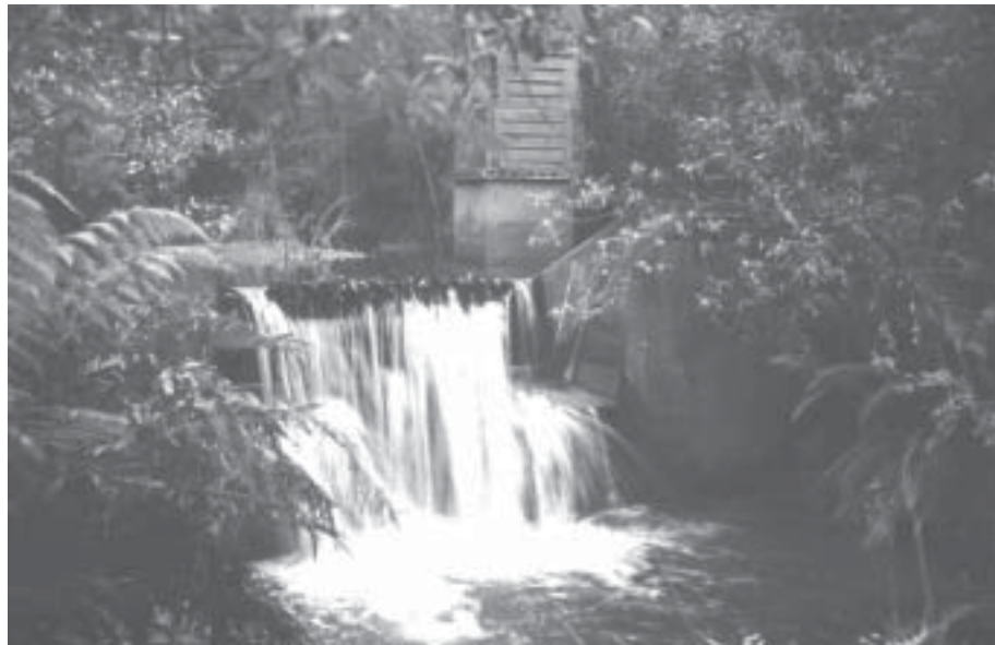
Figure 4. Lees Creek weir after augmentation with metal grill.
