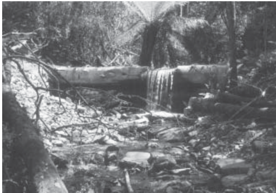
Figure 6. Constructed barrier on Godfrey Creek.
