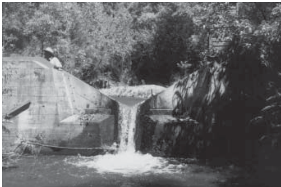
Figure 3. Lees Creek weir before augmentation.
