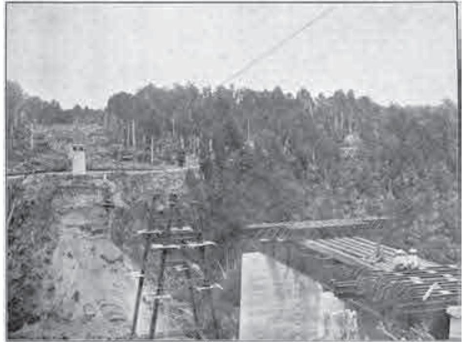
The main trunk line between Wellington and Auckland was officially opened by Prime Minister Joseph Ward on 6 November 1908. It was bounded by several scenic reserves as well as much land that is now part of the conservation estate. AJHR: Weekly Press, AJHR 1907, C6, opp. p. 9;
