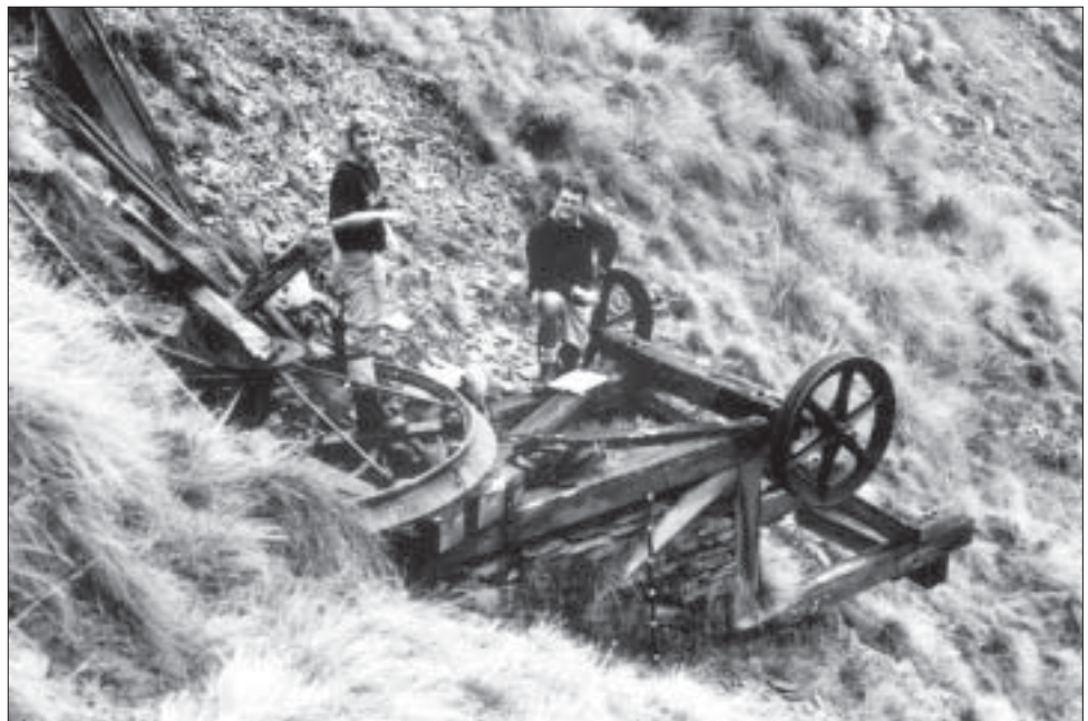
Figure 20. The Homeward Bound aerial cableway top return wheel. Photo: K. Jones, Department of Conservation, Wellington
