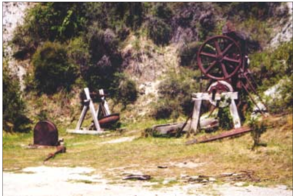
Figure 22. Anderson's Battery site. Photo: P. Petchey.
