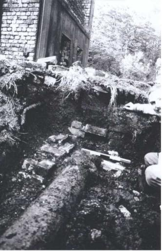
Photo 5: Brick corbelling covering steam pipes returning to condenser.
