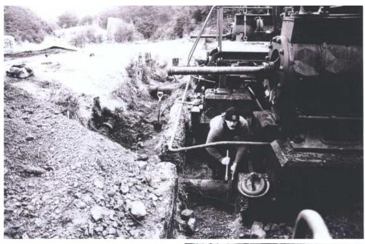
Photo 4: Removing steam pipes.
