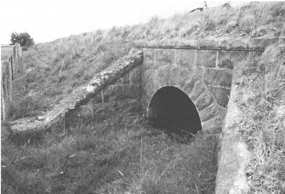
Figure 6 Some fine culverts built with Waipiata basalt, uniquely brought to course. Upper: Open culverts (69.32 and 75.38). Below: An arched culvert (74.67) and a square culvert (65.65).
