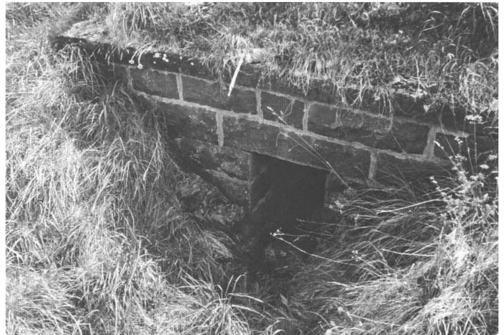
Figure 6 Some fine culverts built with Waipiata basalt, uniquely brought to course. Upper: Open culverts (69.32 and 75.38). Below: An arched culvert (74.67) and a square culvert (65.65).
