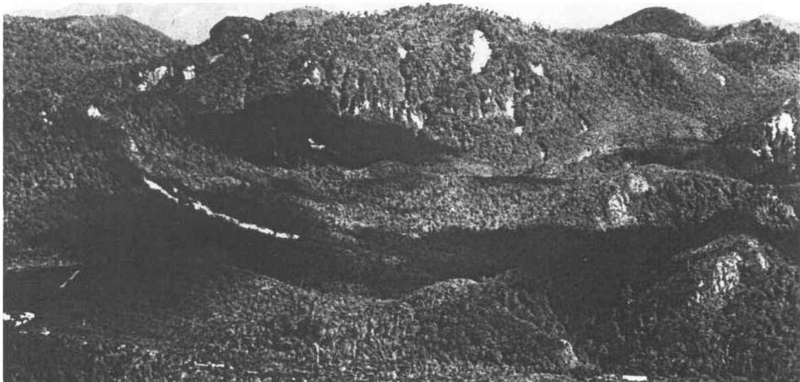
PLATE 3: SHOWING THE 'HIGH POINT', SADDLE, RIDGE LINE AND SLIPS.
