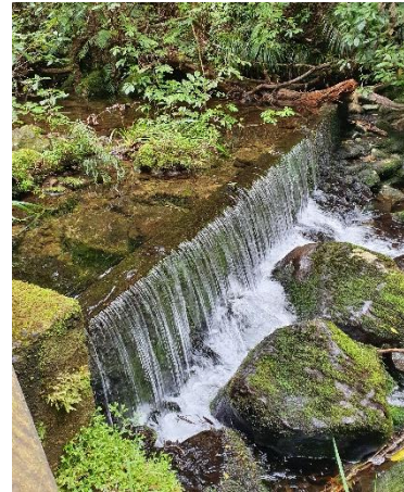
Left: Flapgates at Havelock in Marlborough are known to be a barrier for whitebait moving upstream. Centre: Sjaan Bowie, DOC senior technical advisor researching how well retrofitted baffles help whitebait move through this culvert on the West Coast. Right: This weir in Puketi Forest would prevent īnanga moving upstream. Photos from left: Sarah Wilcox, Nixie Boddy, Sjaan Bowie DOC
