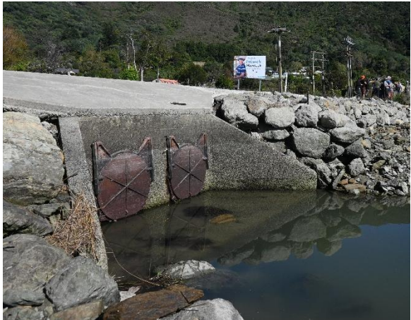
Left: Flapgates at Havelock in Marlborough are known to be a barrier for whitebait moving upstream. Centre: Sjaan Bowie, DOC senior technical advisor researching how well retrofitted baffles help whitebait move through this culvert on the West Coast. Right: This weir in Puketi Forest would prevent īnanga moving upstream. Photos from left: Sarah Wilcox, Nixie Boddy, Sjaan Bowie DOC
