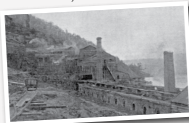
A truck brings fireclay from the St Kilda mine (note bins in background) past the coke ovens to the back of the pug mill, c. 1913.
