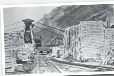
An L wagon transports fire clay goods and coke to the bridge turntable.
