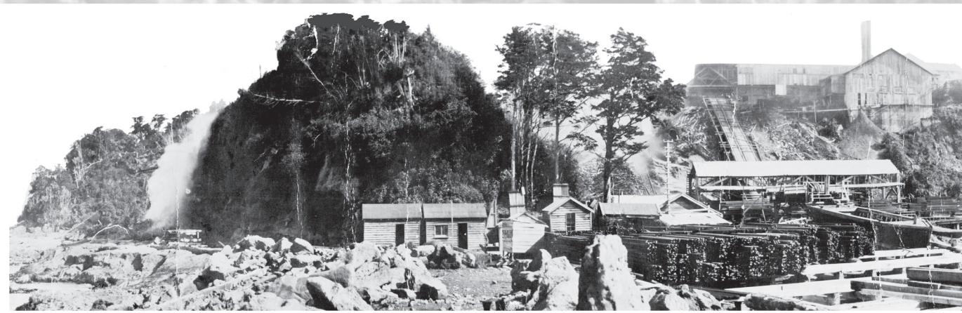
Port Craig sawmill and timber stack. (Photo: Hocken Library)
