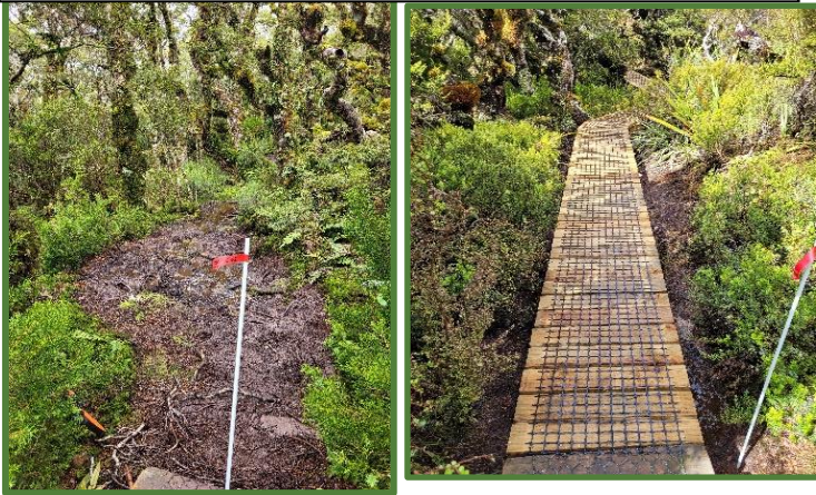
Above/Below: Two examples of upgrade work (before/ during, after) to improve track conditions underfoot.
