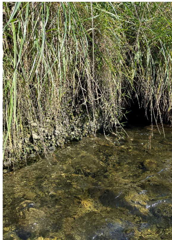
Figure 3-12: Undercut banks near Mazengarb Stream
