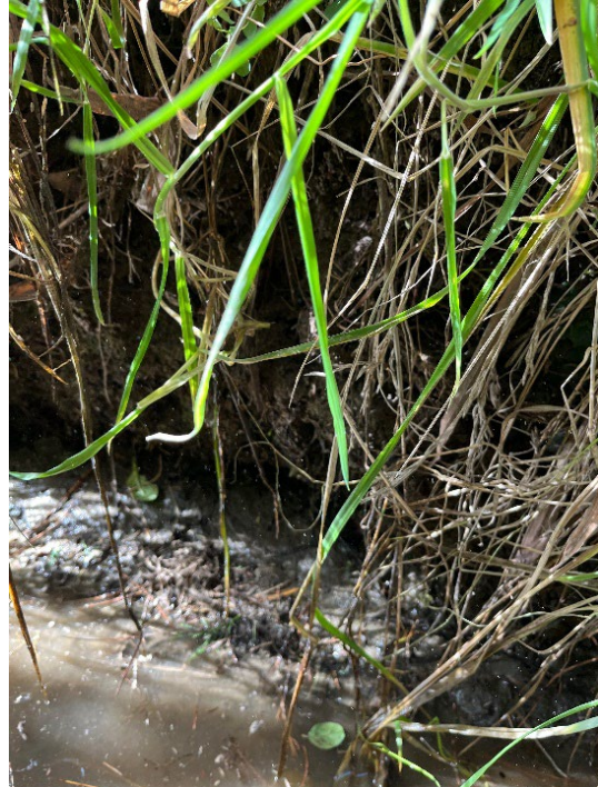
Figure 3-10: Undercut on true right bank below oxbow
