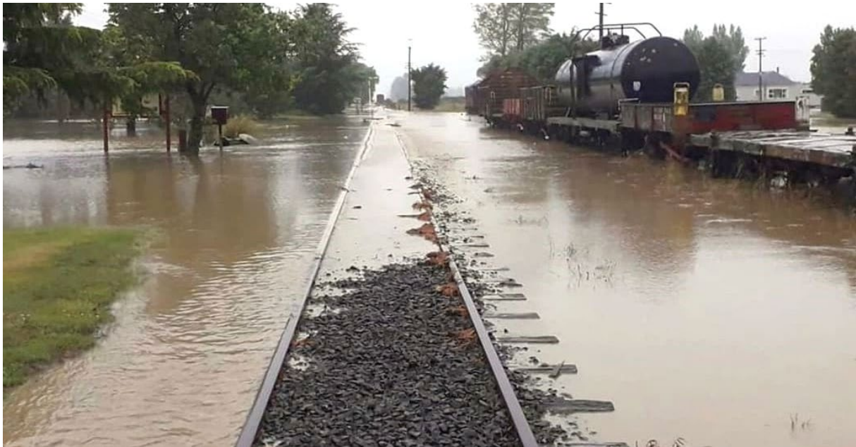
Figure 4-6 Floodwaters in Middlemarch, January 2021. Source: RNZ, https://www.rnz.co.nz/news/national/433989/severe-weather-eases-over-otago
