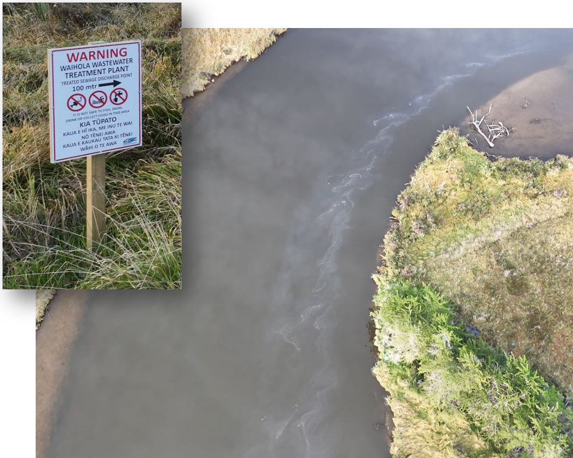
Figure 7-7 Discharge from the Waihora Wastewater Treatment Plant, in the Waipōuri River in April 2023. Inset: warning sign near the discharge point (Source: GHC)
