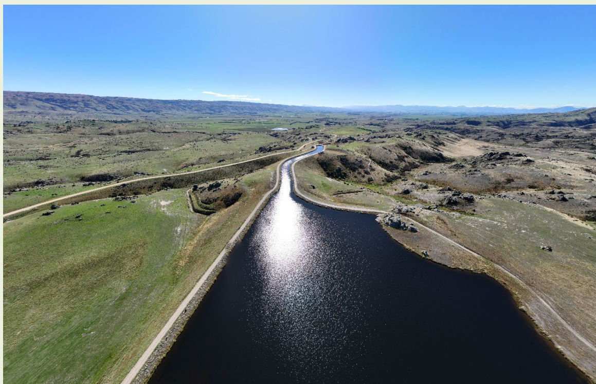
Water storage and canal above the Maniototo Plain, at Stonehenge (Source: GHC)
