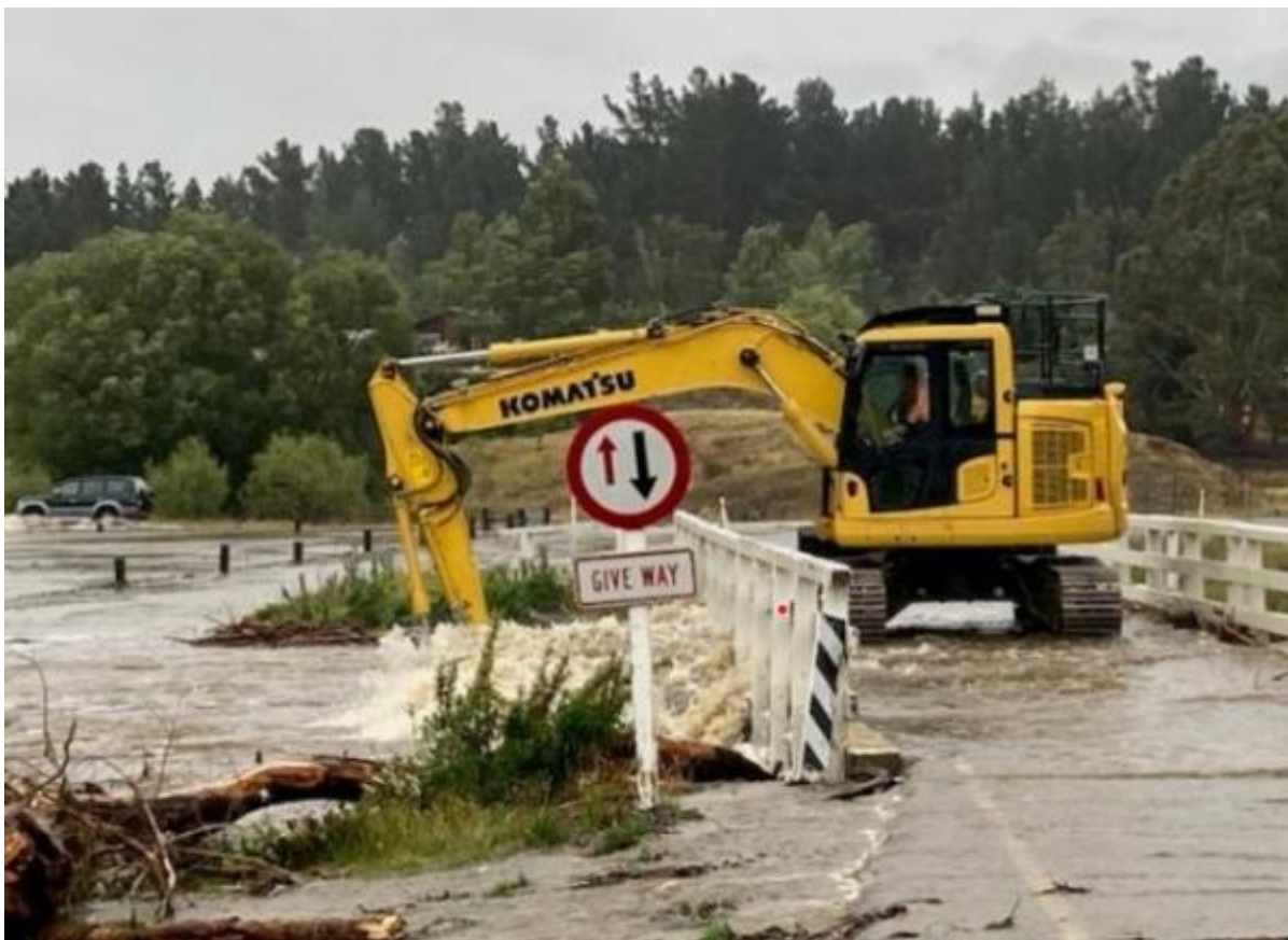
Pātearoa township bridge being cleared of debris after flooding in the Māniatoto in January 2021 (Source: Central Otago District Council/Fulton Hogan/Otago Daily Times)
