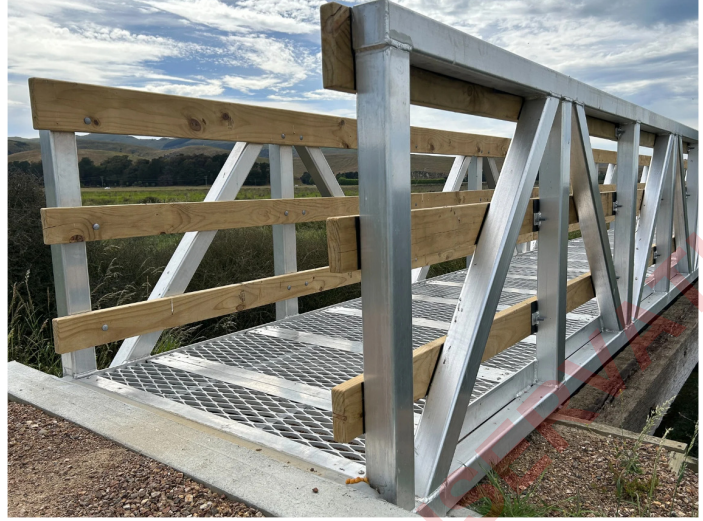
Figure 17 – Aluminium pedestrian bridge with timber railing to improve the aesthetic. (Source: Monkeytoe website).
