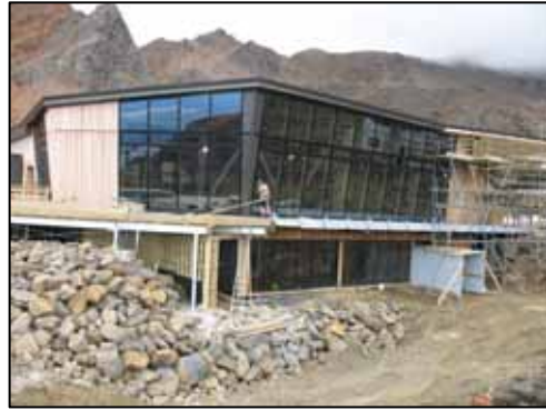
Finishing touches to the newly constructed Knoll Ridge Café Photo: DOC
