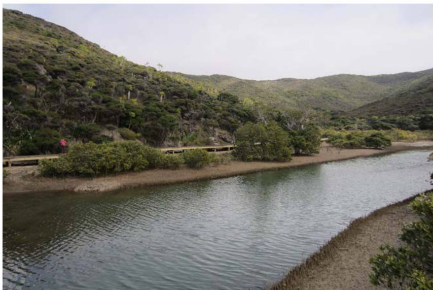
View from new bridge at Tapotupotu
