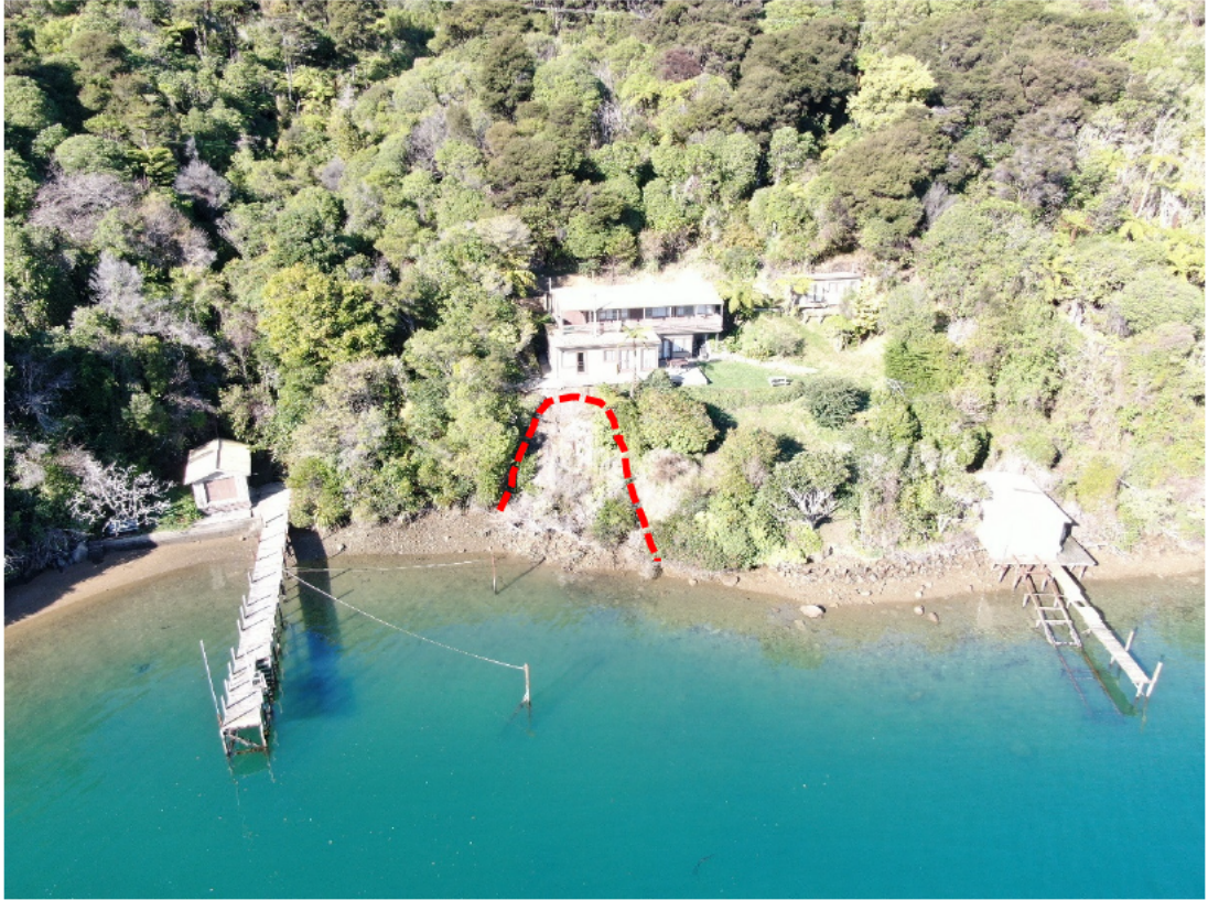
Figure 2: Drone image of the property and landslide
