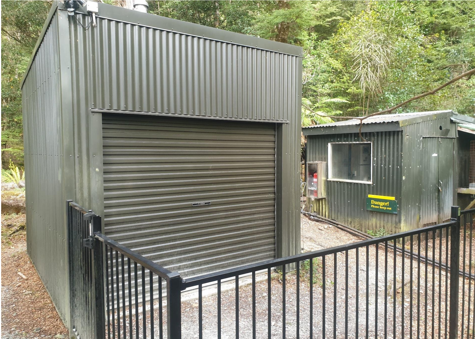
Figure 43. Photo of new generator shed with old generator shed in the background
