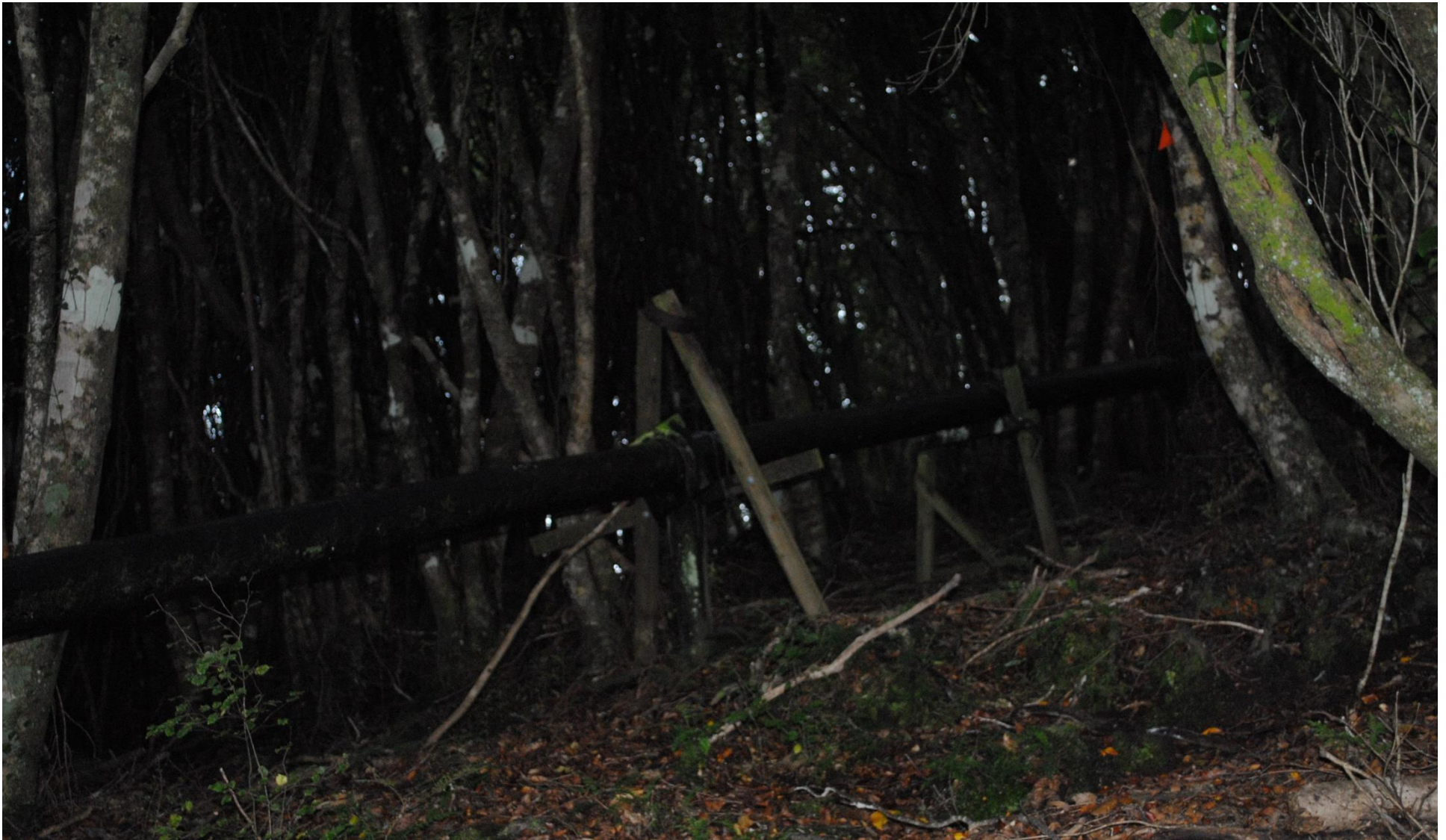
Figure 35. Photo of pipeline including support structures
