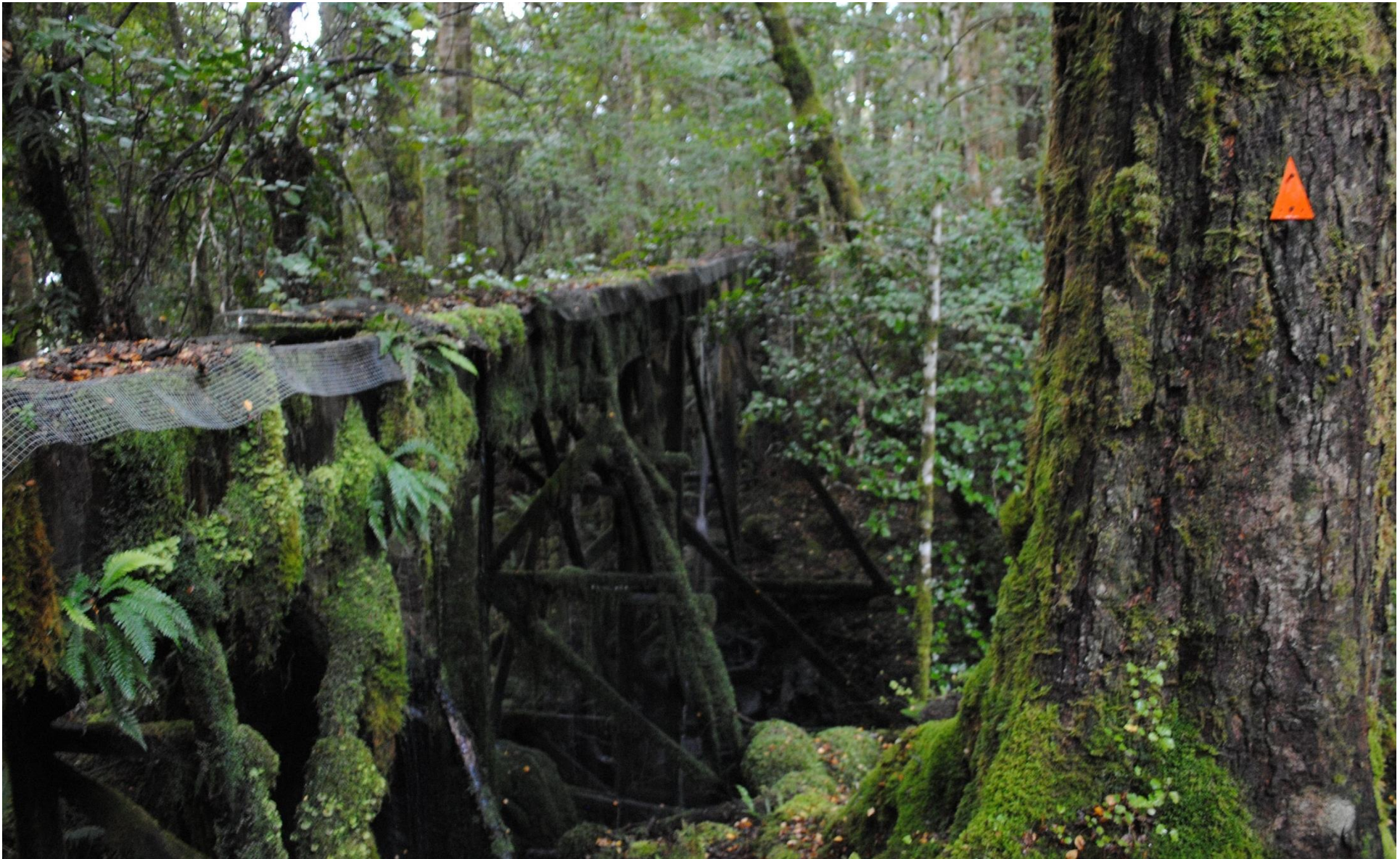
Figure 32. Photo of aqueduct race / screens / structures carrying water to the start of the hydro pipeline
