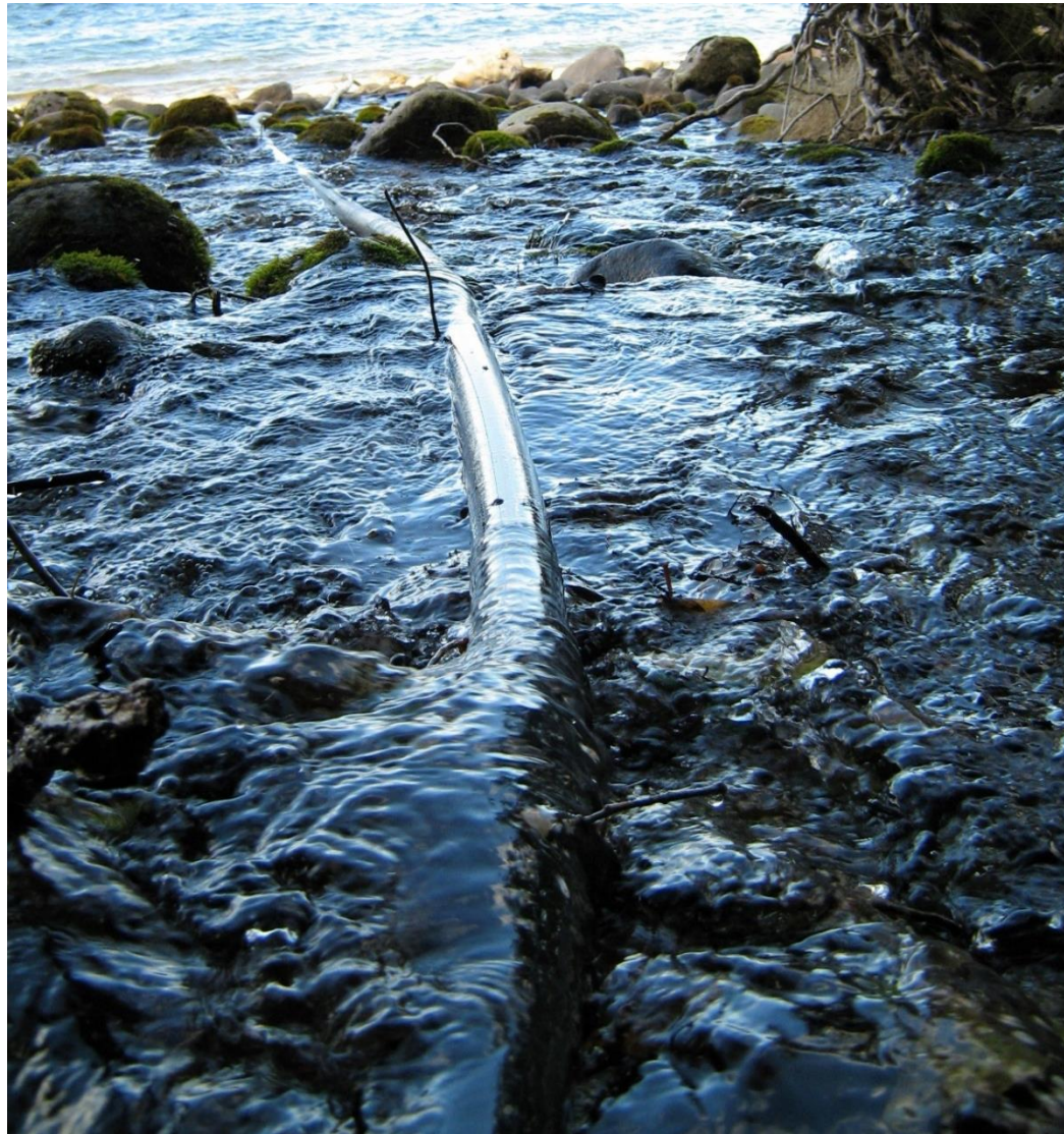
Figure 46. Photo of pipeline into the lake for water take
