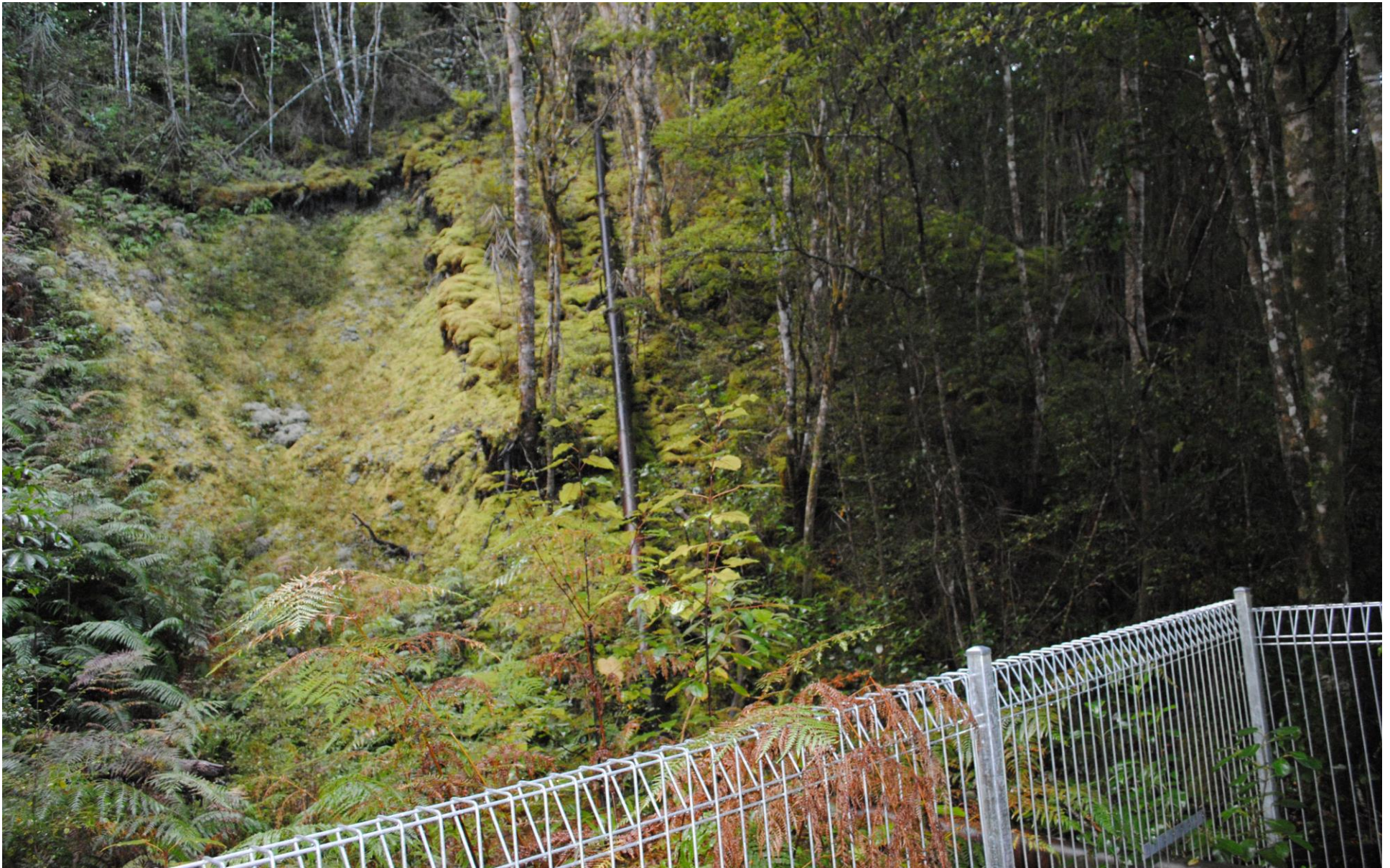
Figure 36. Photo of the last section of the pipeline before the hydro
