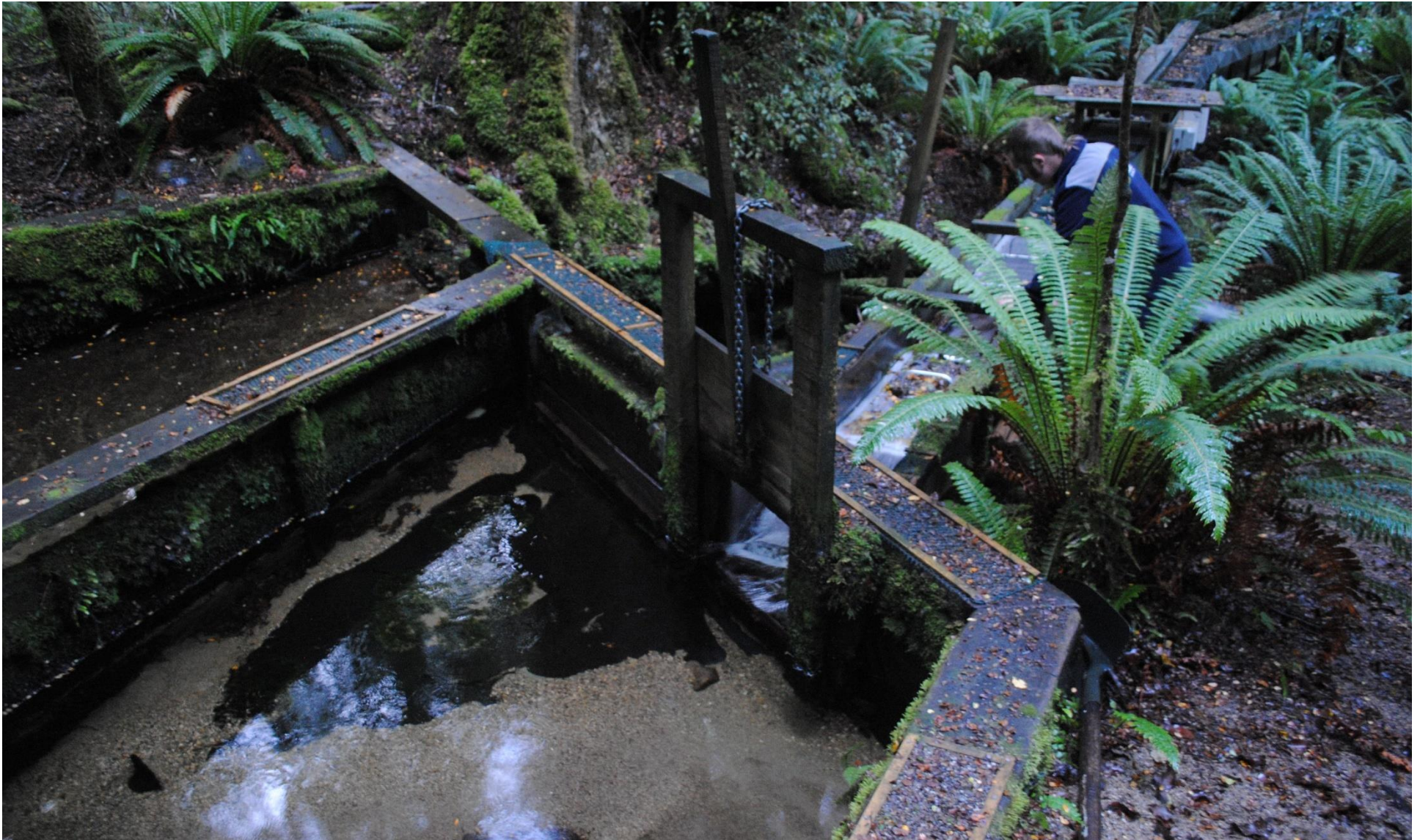
Figure 31. Photo of the Hydro 'dam' and intake
