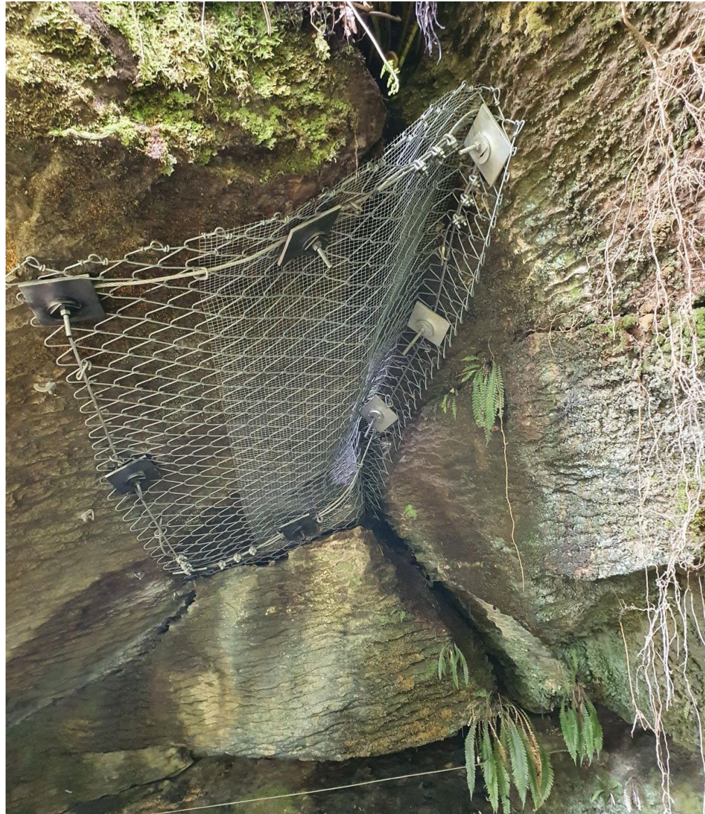
Figure 72. Cave entrance protection structures
