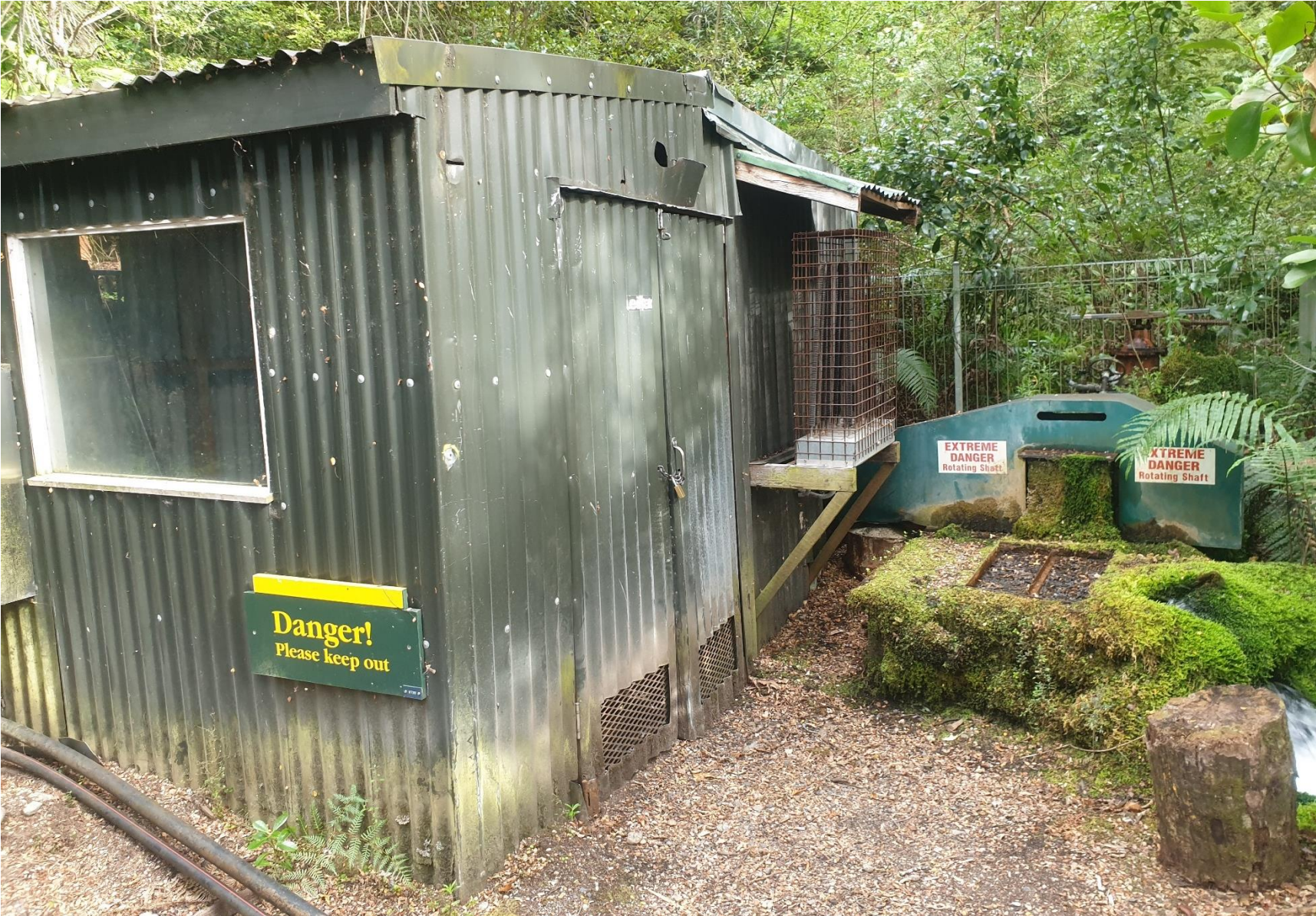
Figure 41. Photo of the Old Generator Shed
