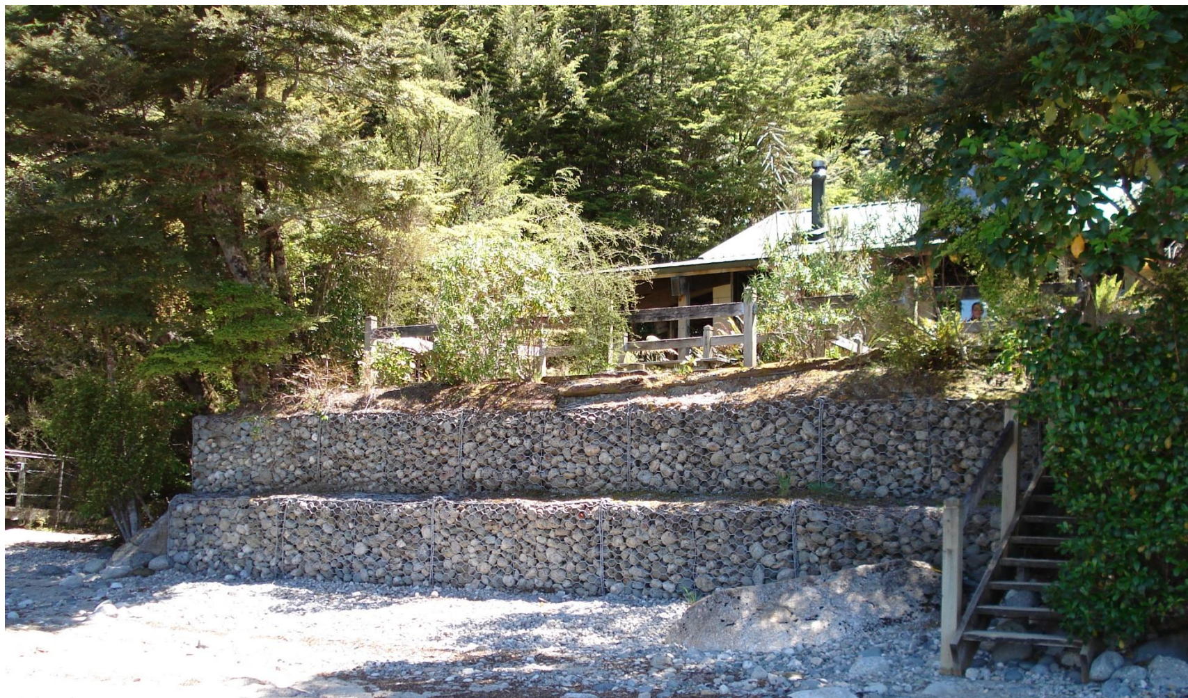
Figure 49. Photo of gabion baskets that support the viewing platform
