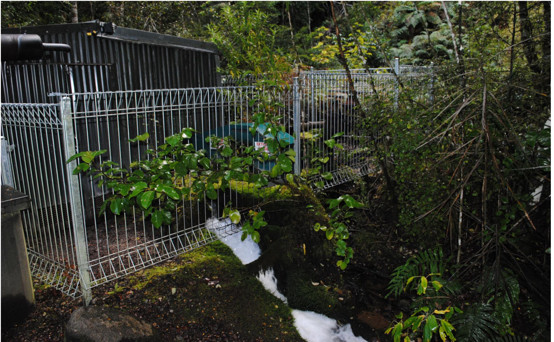
Figure 39. Photo of old generator shed, Hydro, and outflow (discharge race) from hydro
