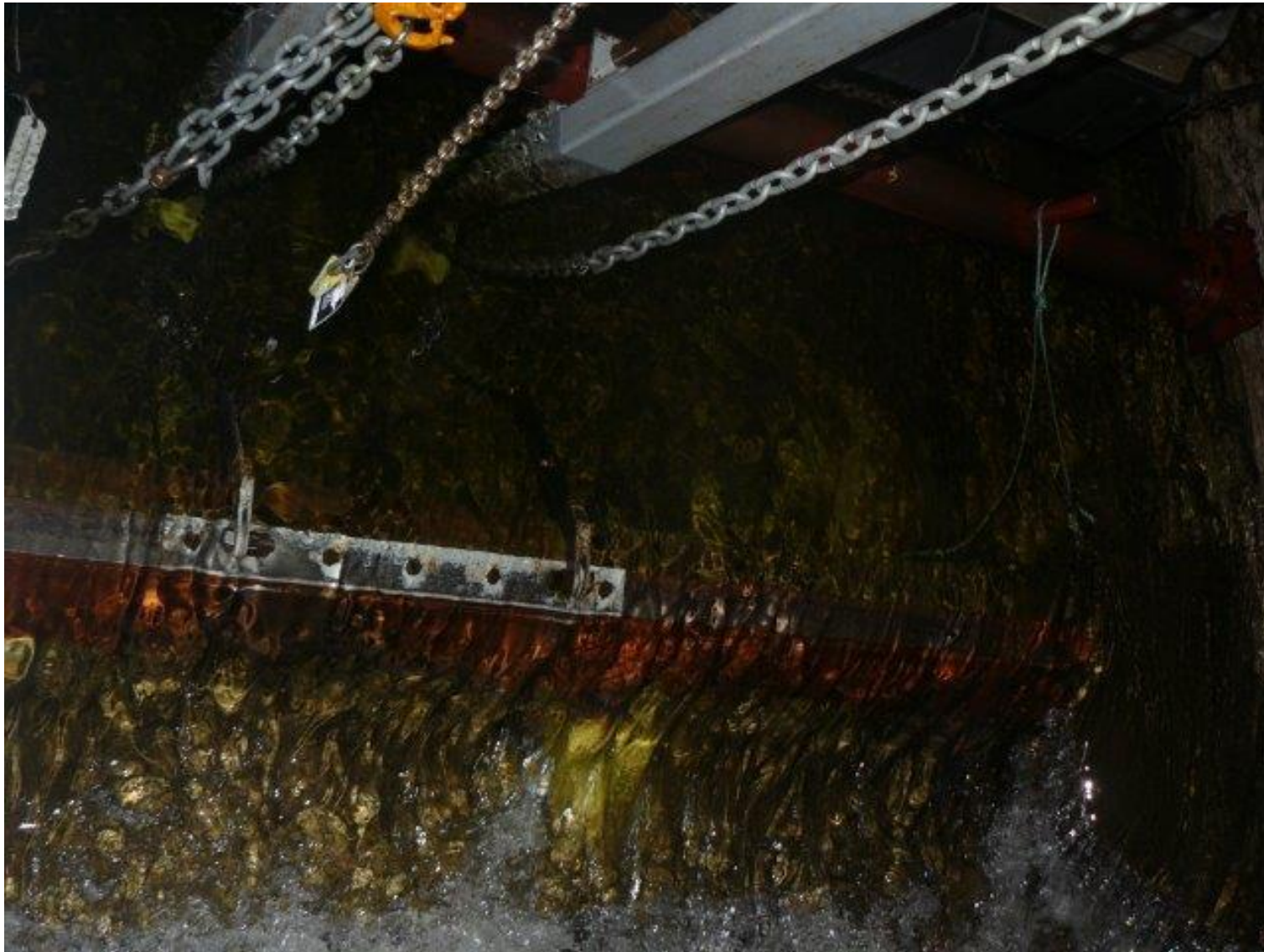
Figure 51. Photo of the dam in the caves which creates the Glow Worm Grotto
