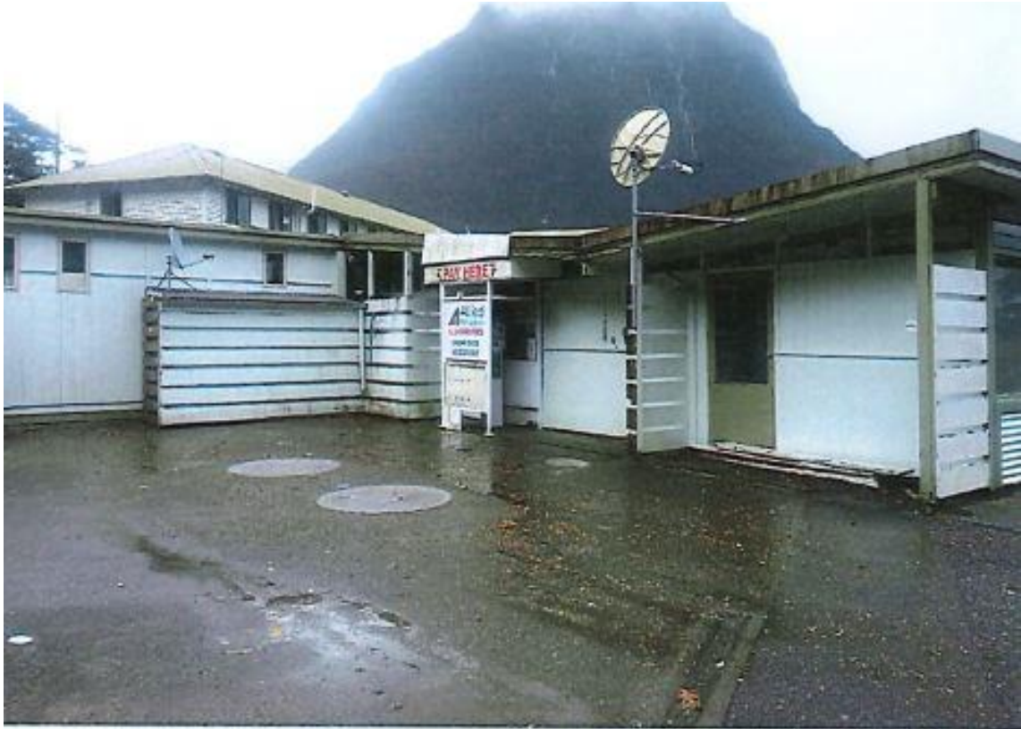
Photograph 2: Photo showing the tank slab (two manholes above the UST). Photo also shows the location of the kiosk.
