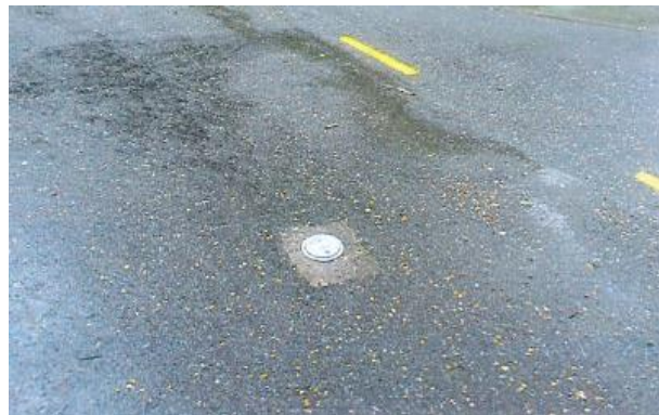
Photograph 3: Photo showing one of the monitoring wells
