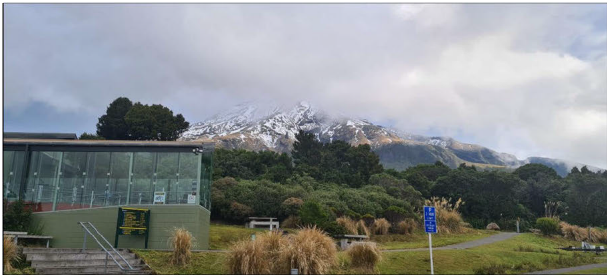
Figure 1: Existing visitor centre
