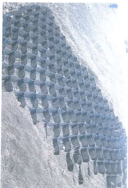
MACCAFERRI GEOWEB - BEAUMONT BRIDGE, MANAKAU CITY http://www.maccferri.com.au/files/Maccaferridemo/04%20beam%20bridge%20steel%20road%20bridge.pdf
