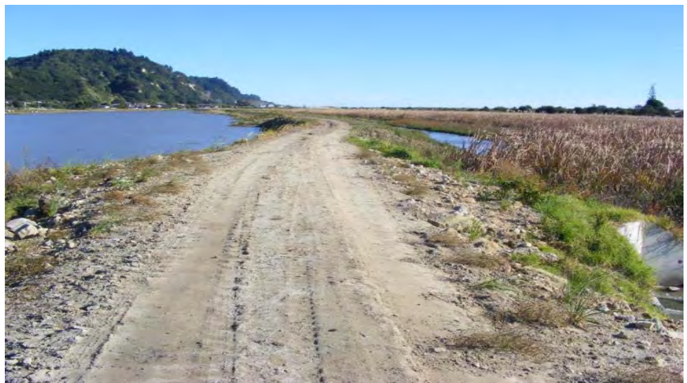
Post completion of rehabilitation works July 2010 (bottom).
