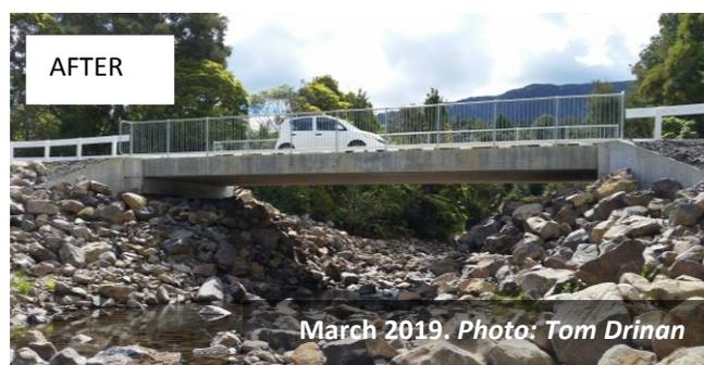
Figure 1. Top – Roadway ford prior to removal. Bottom – Single-span bridge replacement.
