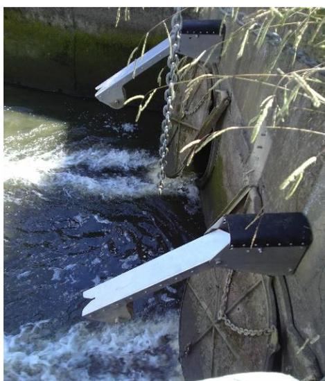
Figure 1. Top-hinged tide-gated culverts at the Awatapu Lagoon with Fish Friendly gate attachments installed (2012. Photo: Kelly Hughes)
