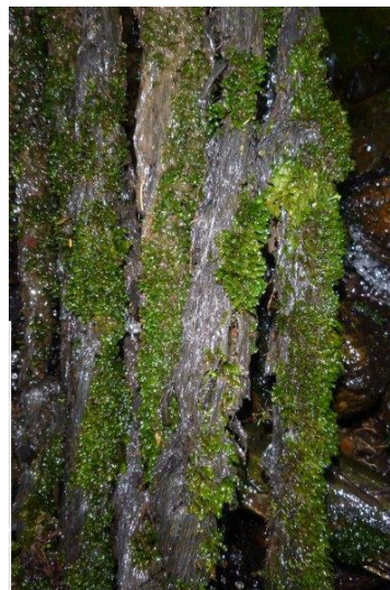
Figure 3. Photos from follow up visits to the perched culvert, showing that the ropes were still in excellent condition and remained taut with biological growth of mosses and filamentous algae covering (2015 and 2019. Photo: Bruno David).
