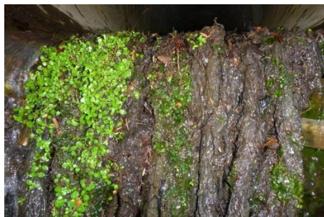
Figure 3. Photos from follow up visits to the perched culvert, showing that the ropes were still in excellent condition and remained taut with biological growth of mosses and filamentous algae covering (2015 and 2019. Photo: Bruno David).
