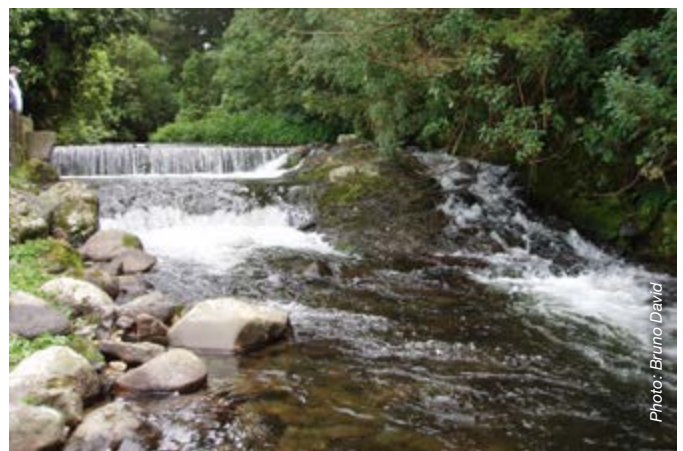
Rock-ramp fishway installed at a weir in Taranaki.
