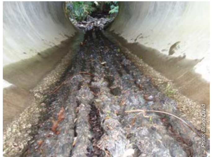
Spat ropes installed in a culvert.
