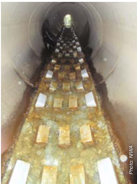
Spoiler baffle sheets installed in a culvert.
