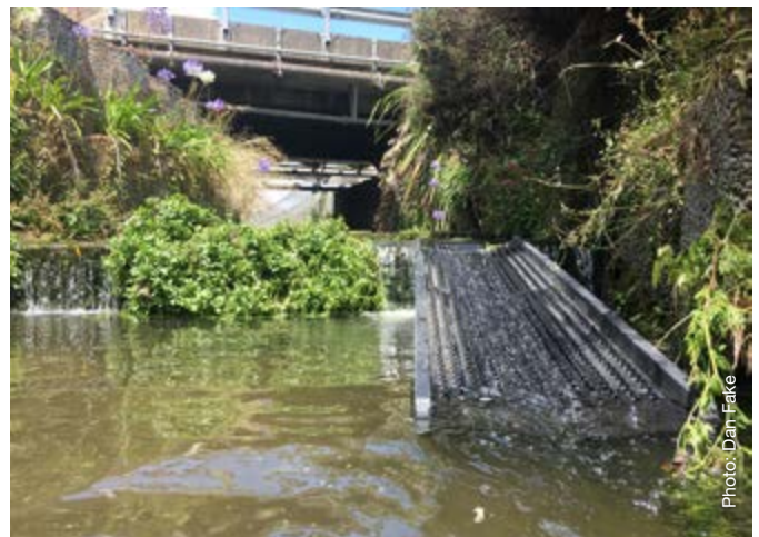
A floating fish ramp installed at a culvert in Hawke's Bay.
