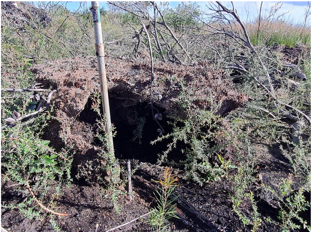
Figure 5. Image taken in May 2023 (about 18 months post-fire) showing a small section of remnant surface about 40 cm above the burnt surface and where the fire has burnt in underneath, potentially resulting in slumping of the surface.
