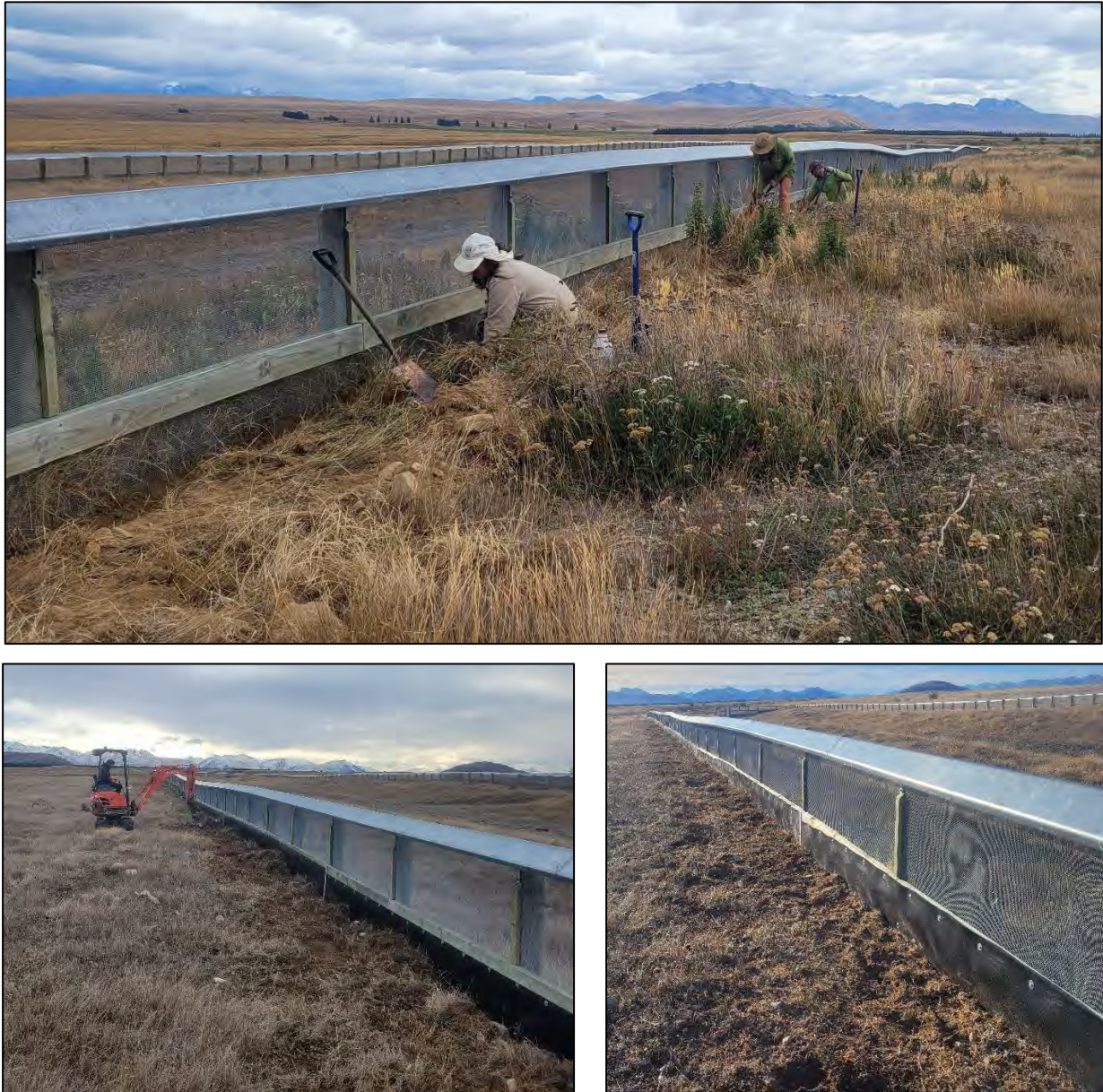
Figure 10. Project River Recovery rangers preparing the existing predator fence for polyethylene membrane installation (top), DOC Twizel back filling soil around the installed membrane (bottom left), the completed membrane installation (bottom right).
