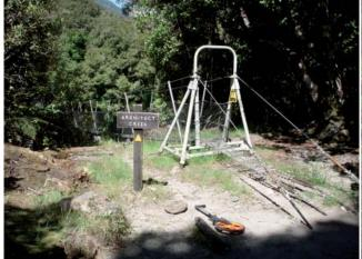
Anchor blocks for original Architects Creek bridge (on the left of and behind the sign) and the 1967 Forest Service design replacement.
