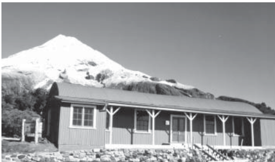
The historic Camphouse following restoration.
