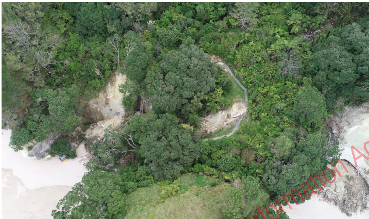
Figure 2.3: Aerial view showing landslides and rockfall around the track.
