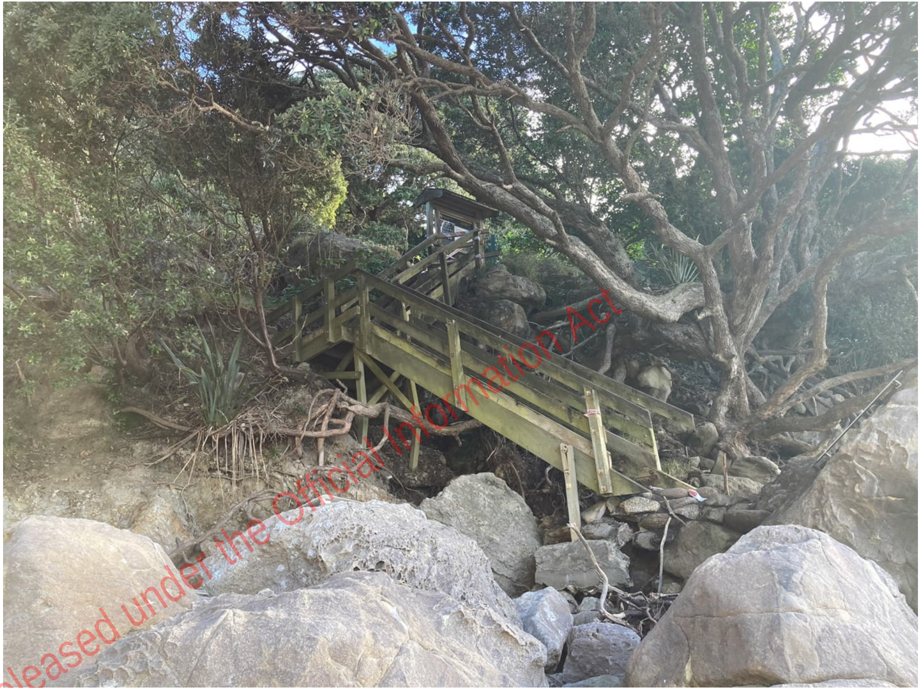
Figure C11 Gemstone Bay stair access
