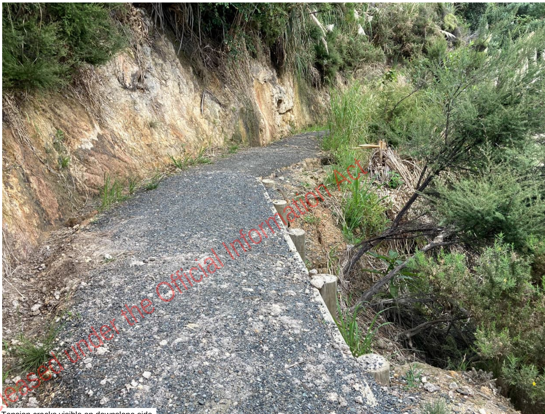
Figure C14 Tension cracks visible on downslope side of Hahei Track
