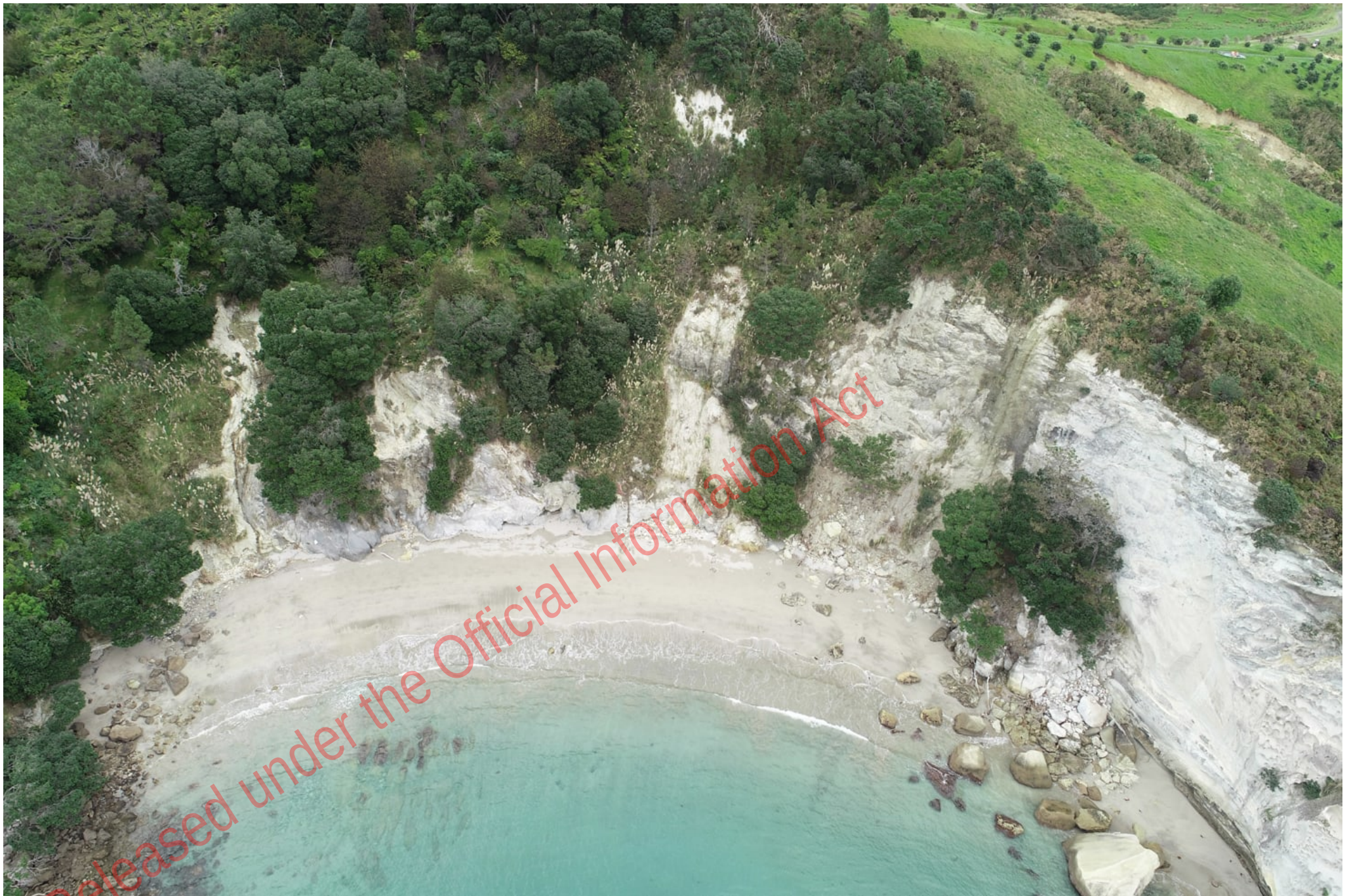
Figure C7 Aerial view of landslides at Stingray Bay
