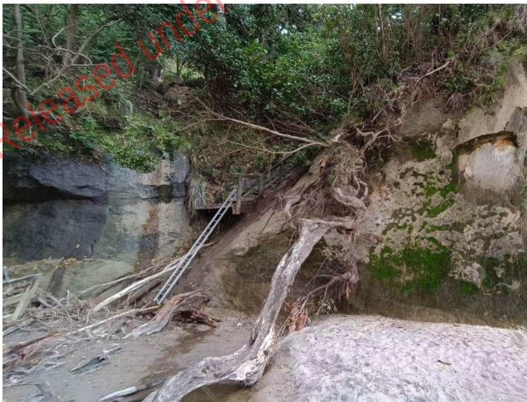
Figure 2.2: 2023 storm event destroyed the stair structure leading to Cathedral Cove Beach.
