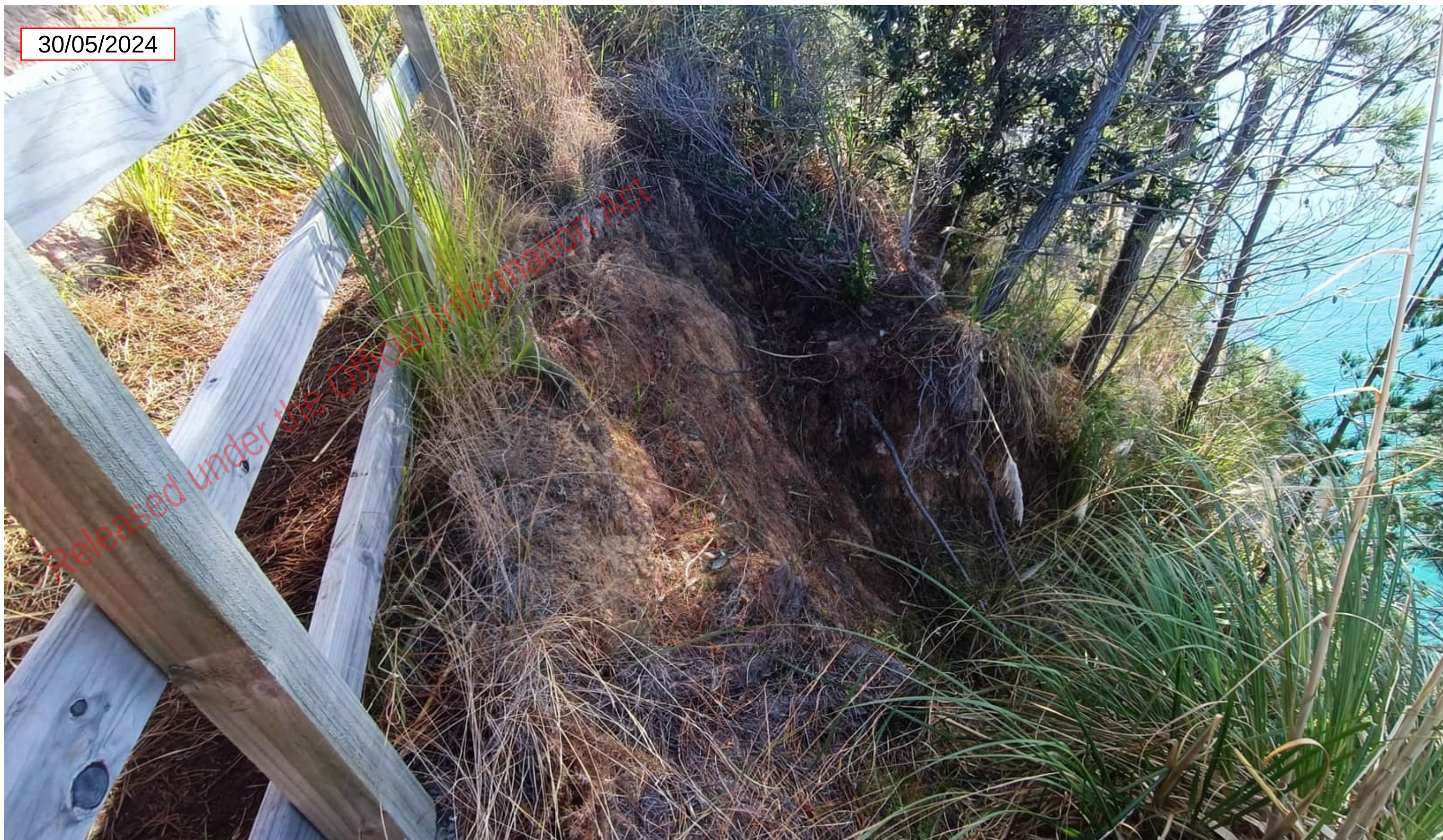
Feature 30 - Translational landslide No new movement observed during May 2024 visit.
