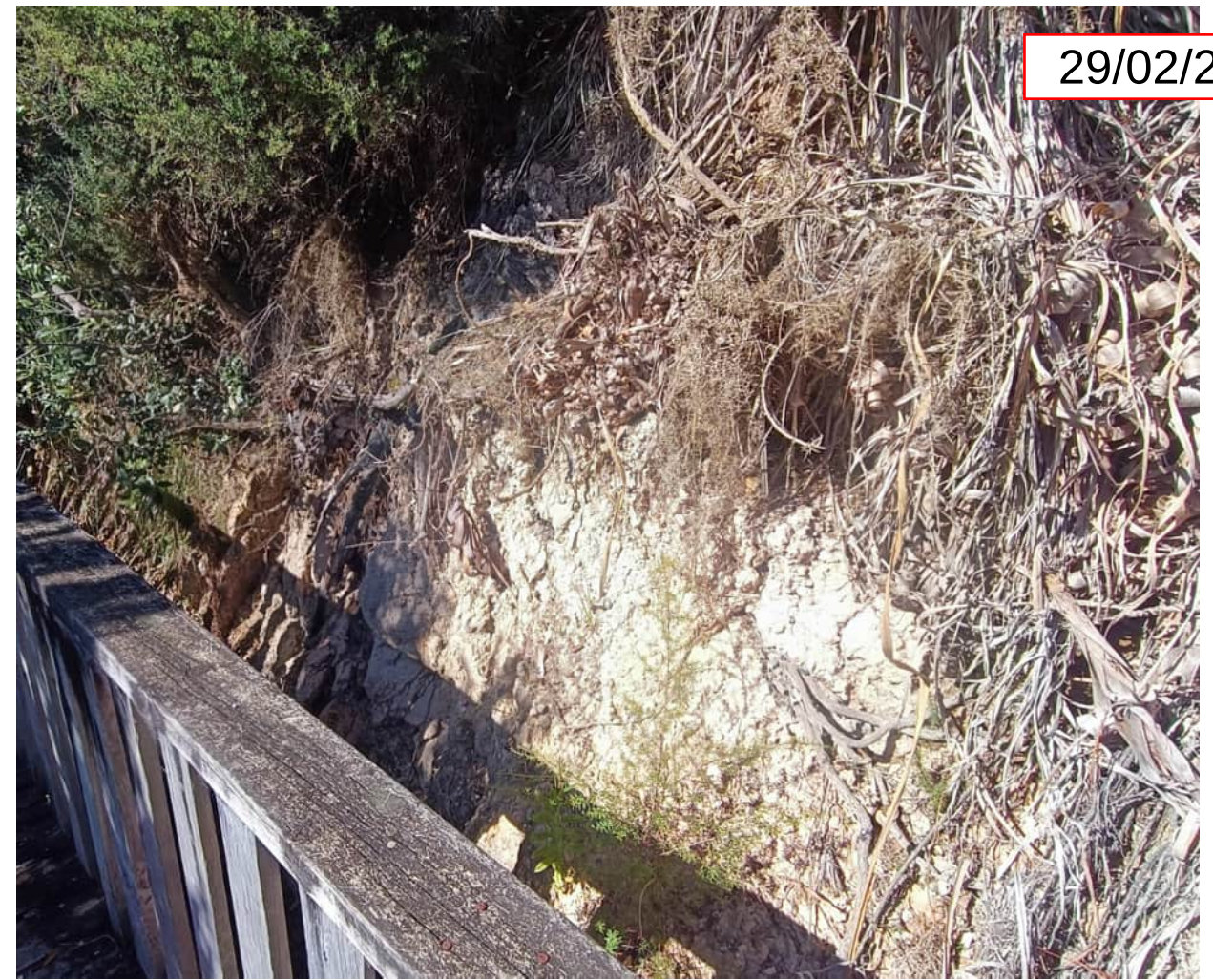
Feature 29 - Historical translational landslide. No new movement of historical landslide. Adjacent slope shows some loose roots
