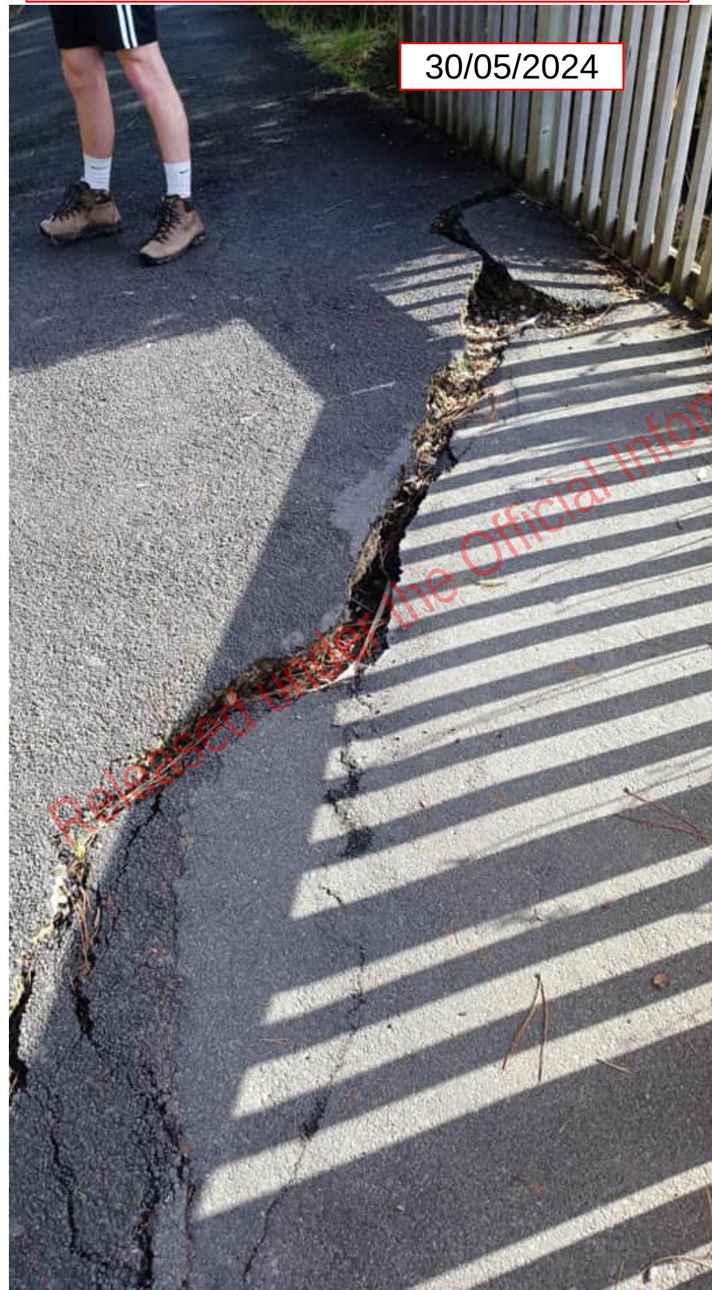
Feature 7 Cont. - Translational landslide Small additional deflection in the scarp observed during May 2024 visit.
