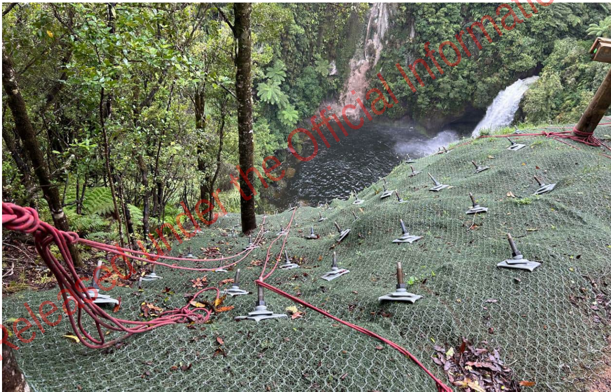
Figure 6.7: Photograph of ground anchorages and Macmat-R mesh during construction at Omanawa Falls. (Source: T+T).
