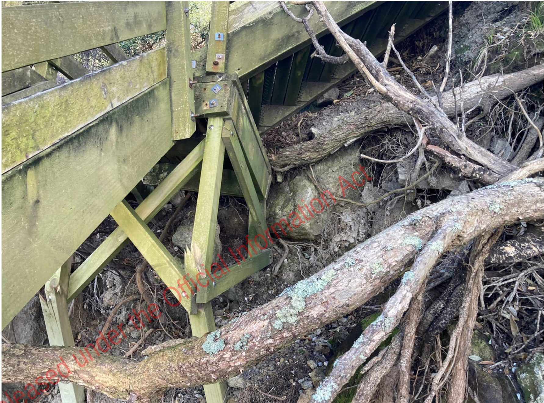
Figure C12 Gemstone Bay stair access damage and scour of loose boulders in slope.
