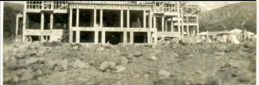
Construction of Chateau Tongariro c. 1929. Source: Manawatu Heritage.
