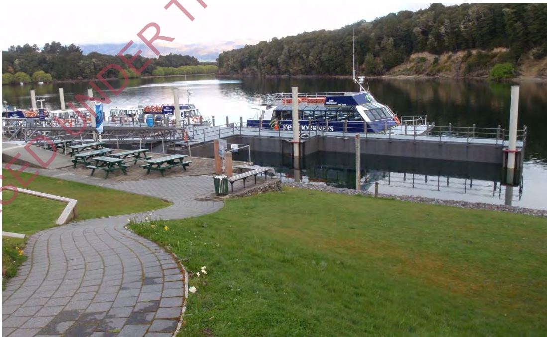
Floating berths for Real Journeys at Pearl Harbour Manapouri 2010
