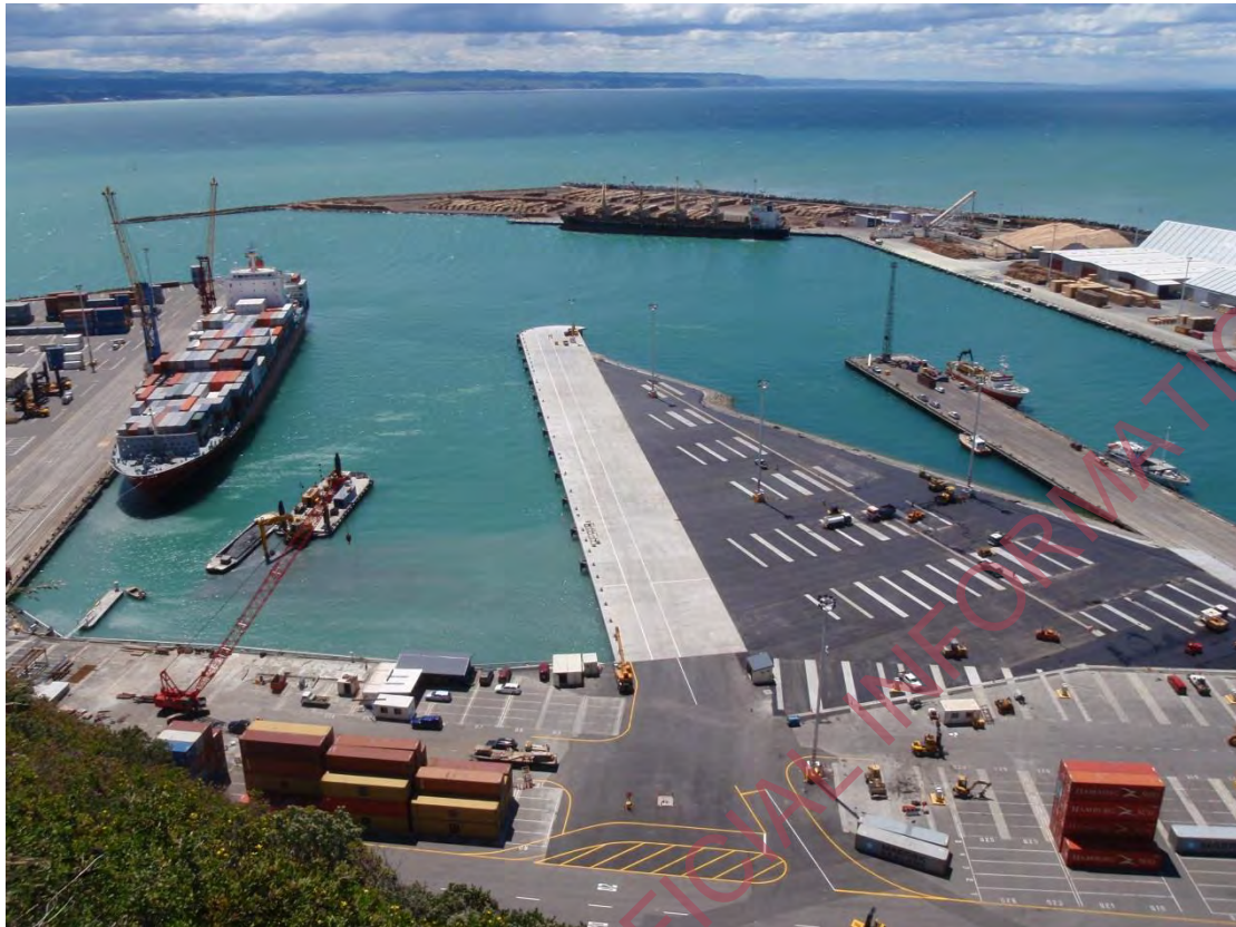
Port of Napier – No 4 Wharf and Reclamation
