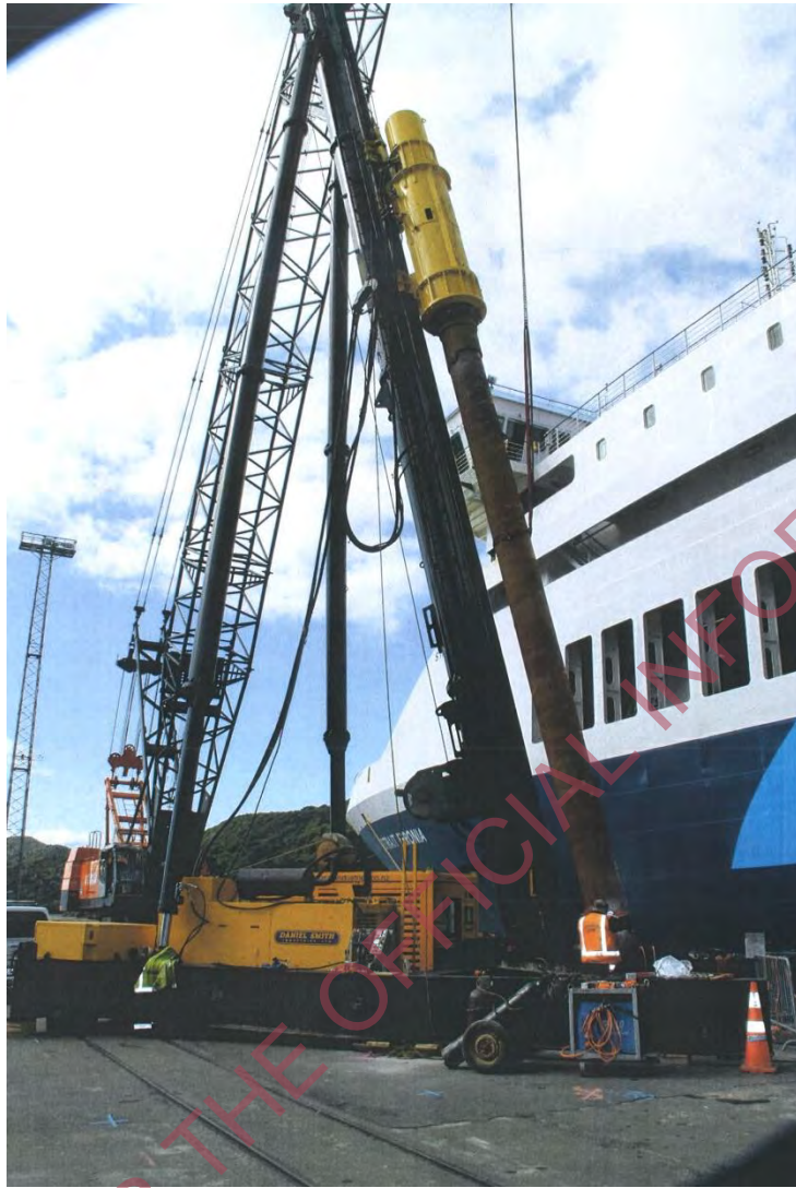
Waitohi Wharf Upgrade 2015
