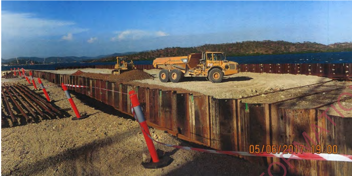
Sheet Piled Quay Wall Port Moresby PNG
