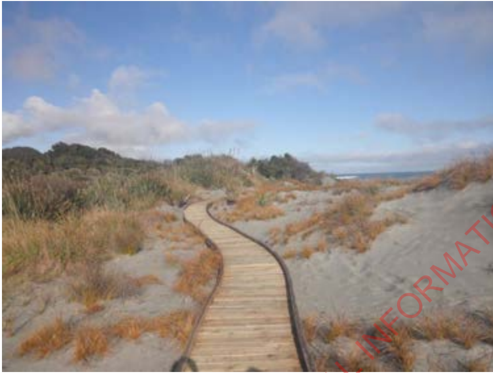
Figure 7: Completed boardwalk at Ship Creek Track.
