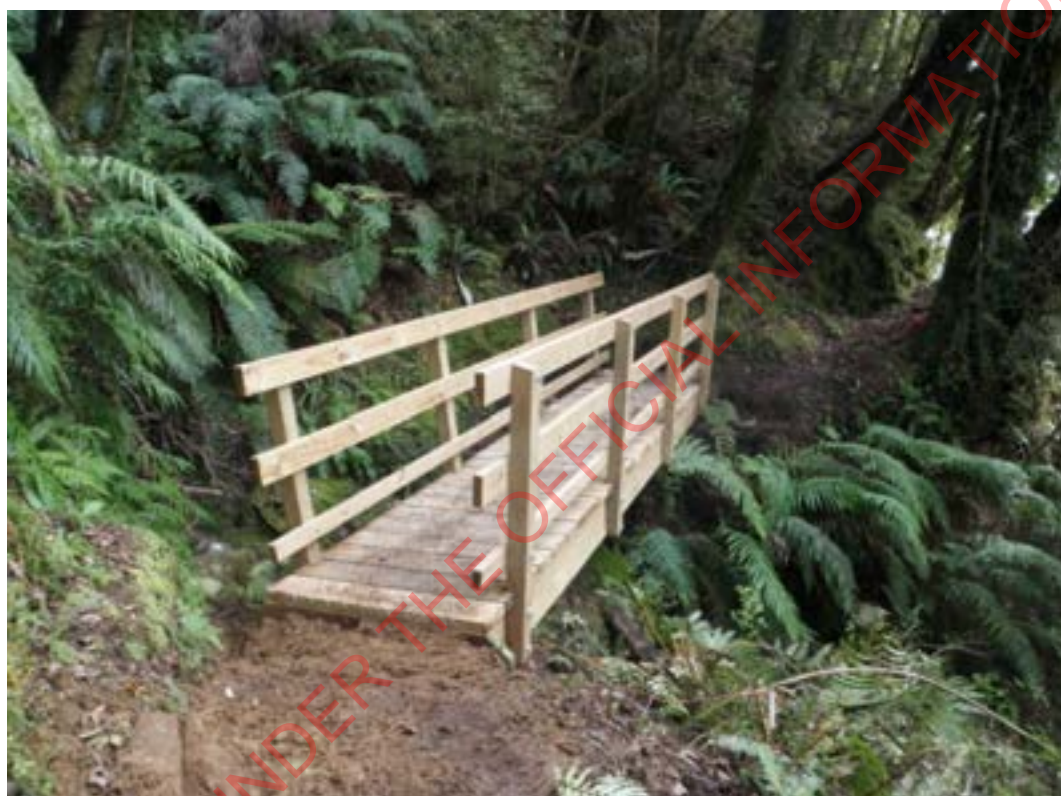
Figure 5: Typical bridge over small water course
