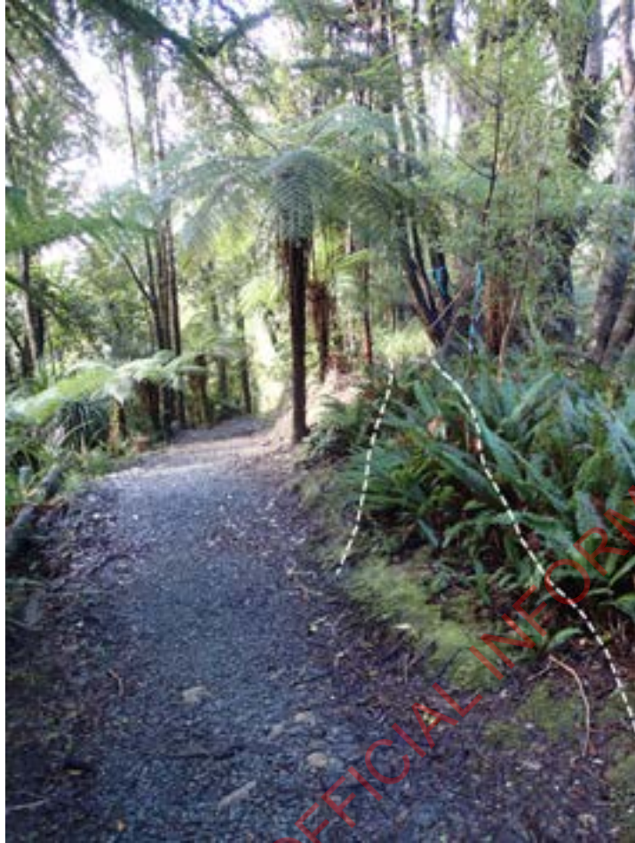
Figure 11. A proposed track junction. A new section of track will be constructed on the left (approximately between the white lines) in order to avoid the steep section of the existing track on the left.
