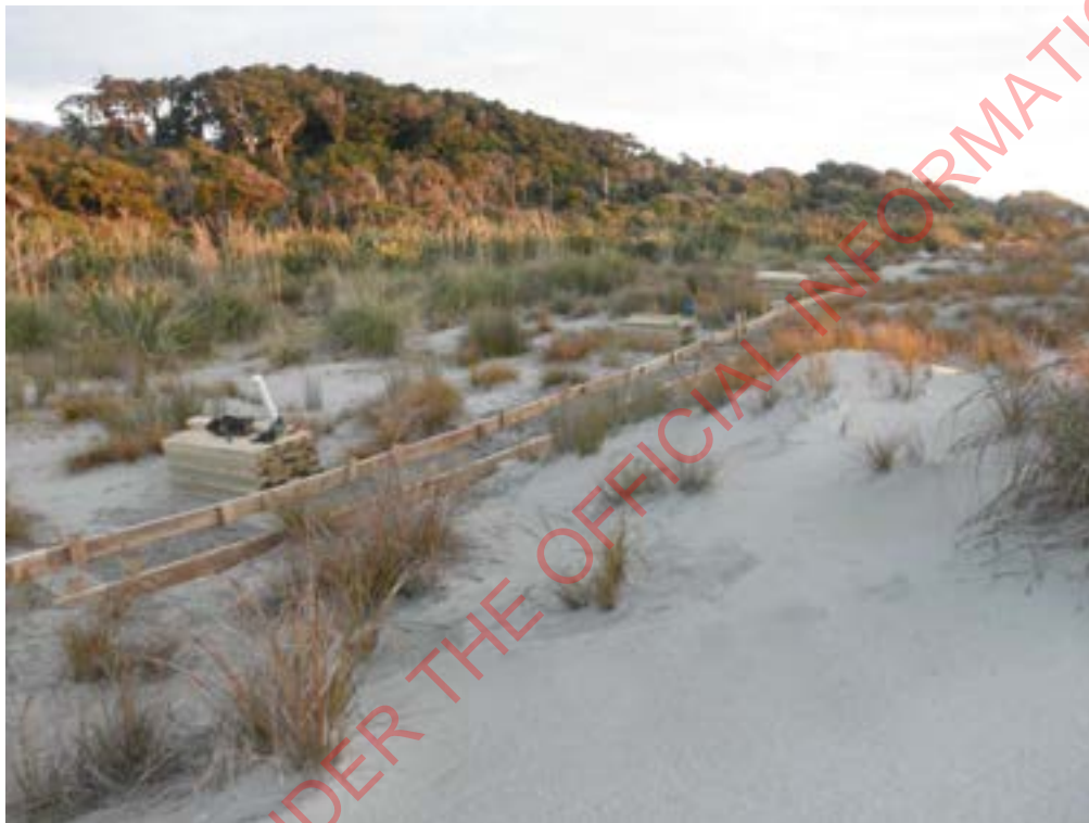
Figure 6: Framing of boardwalk, and timber supplies at Ship Creek Track.
