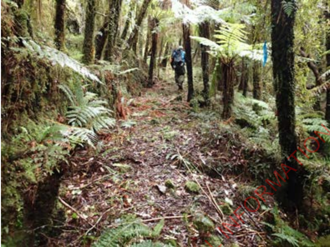
Figure 13. A section of benched track.
