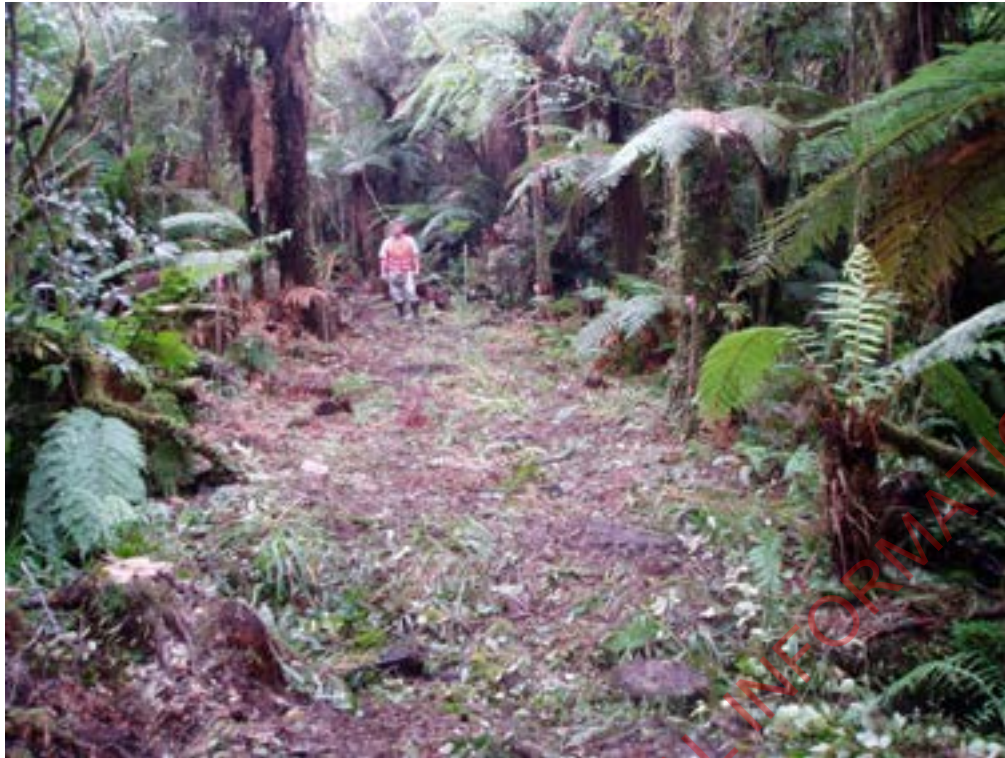
Figure 10: Stage One - Clearance of vegetation for the path.
