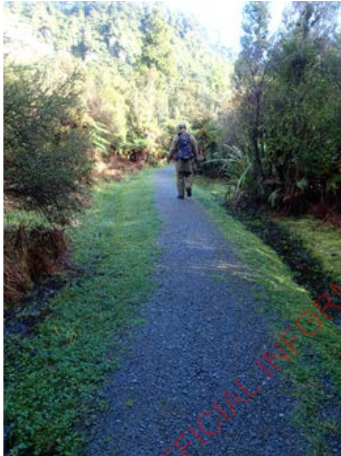
Figure 7. A section of the lower track, near the Punakaiki River, showing the original raised track with drains on either side.
