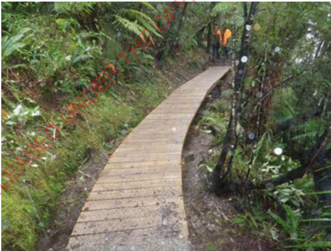
Figure 8: Boardwalk as constructed through a forested landscape.
