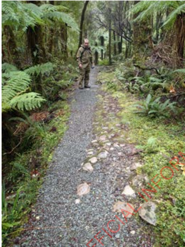
Figure 8. Original track base course (right) next to more modern crushed metal track surface.
