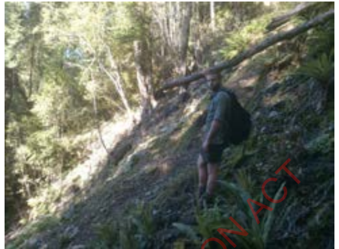
Figure 10: There are a number of small slips in the lower Pike Valley. Potential erosion issues exist but these will be easy to manage with sympathetic track profile setup and execution.
