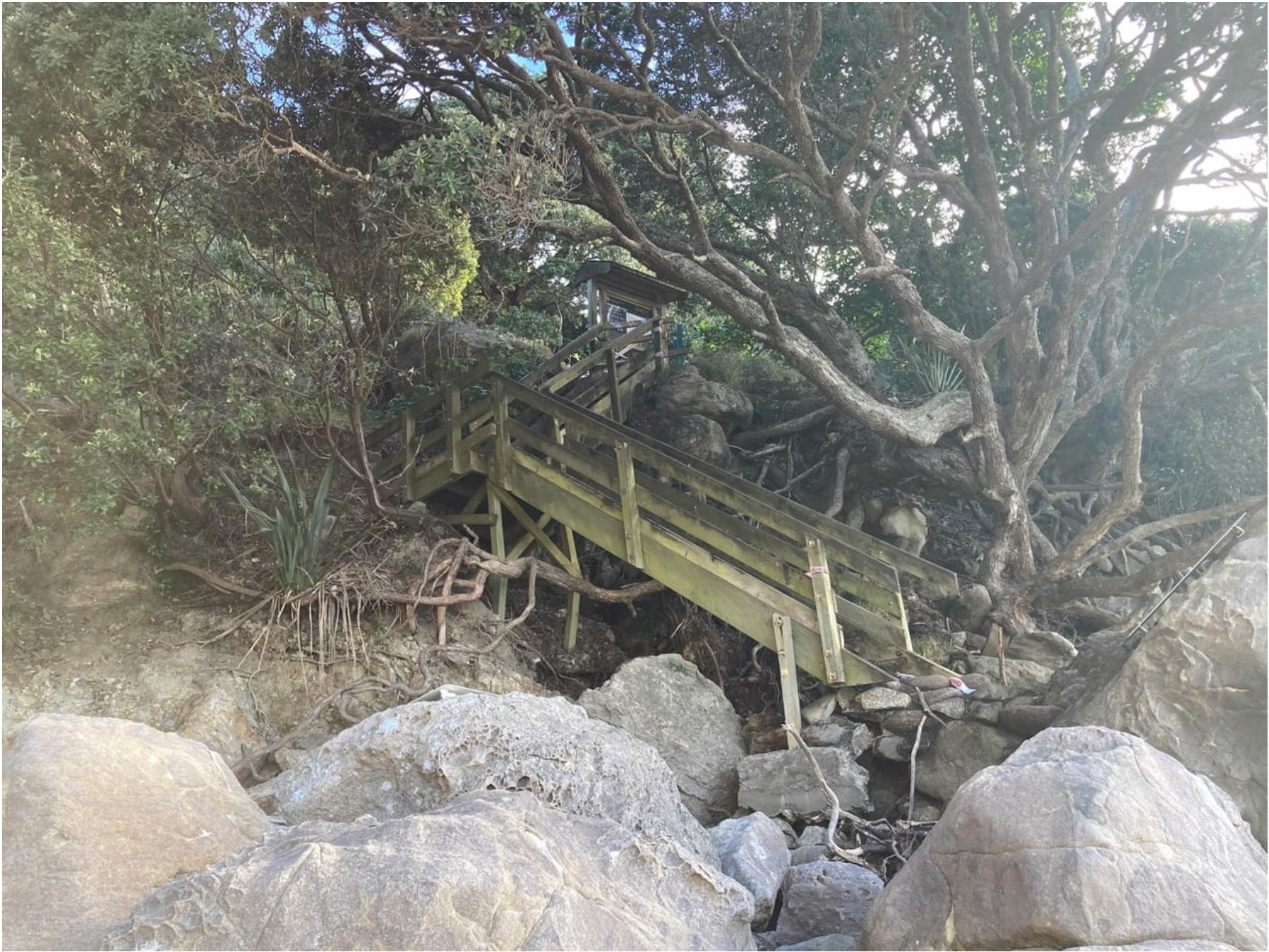
Figure C11 Gemstone Bay stair access
