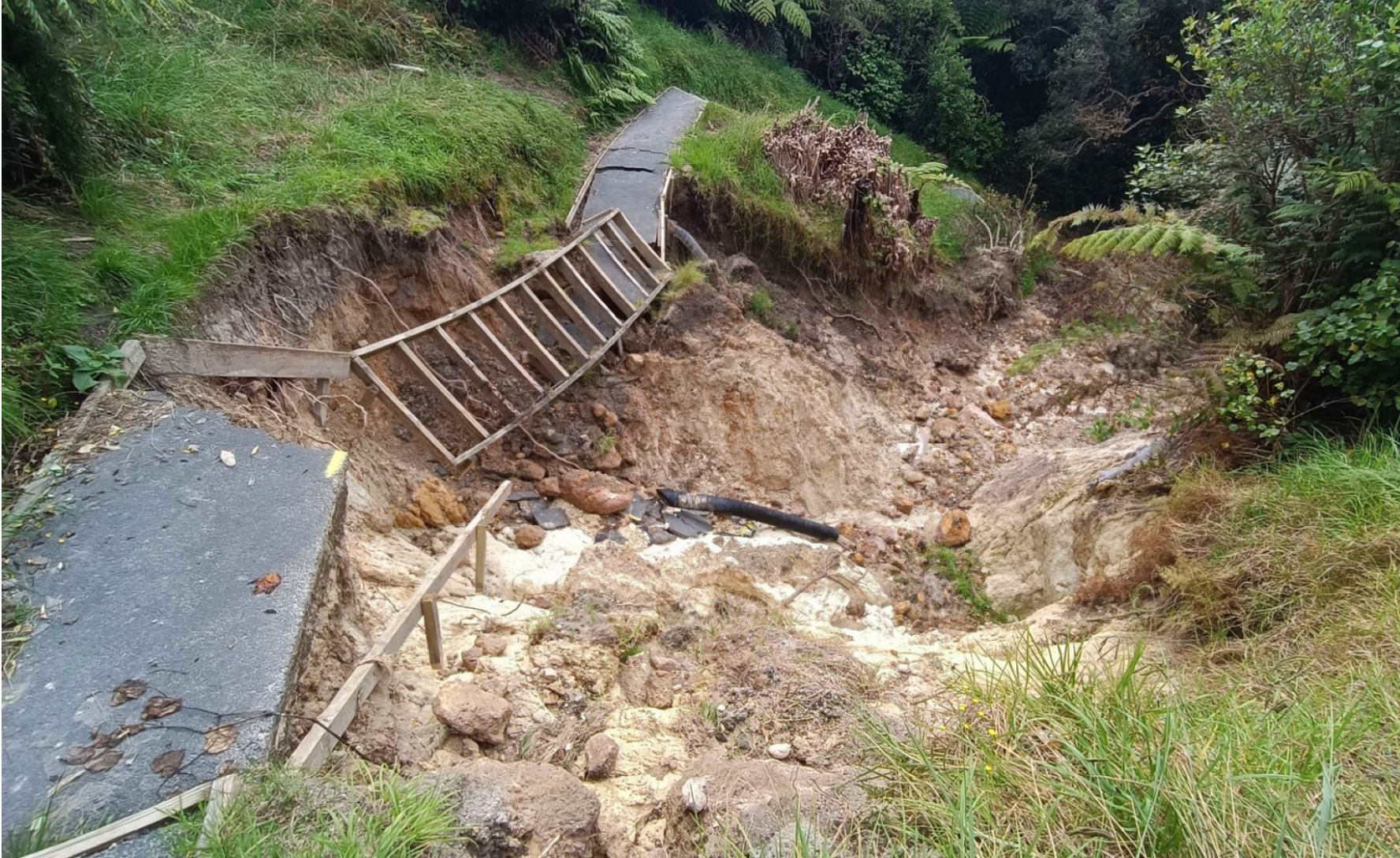
Figure 10.1 Cathedral Cove lower track landslide damage.
