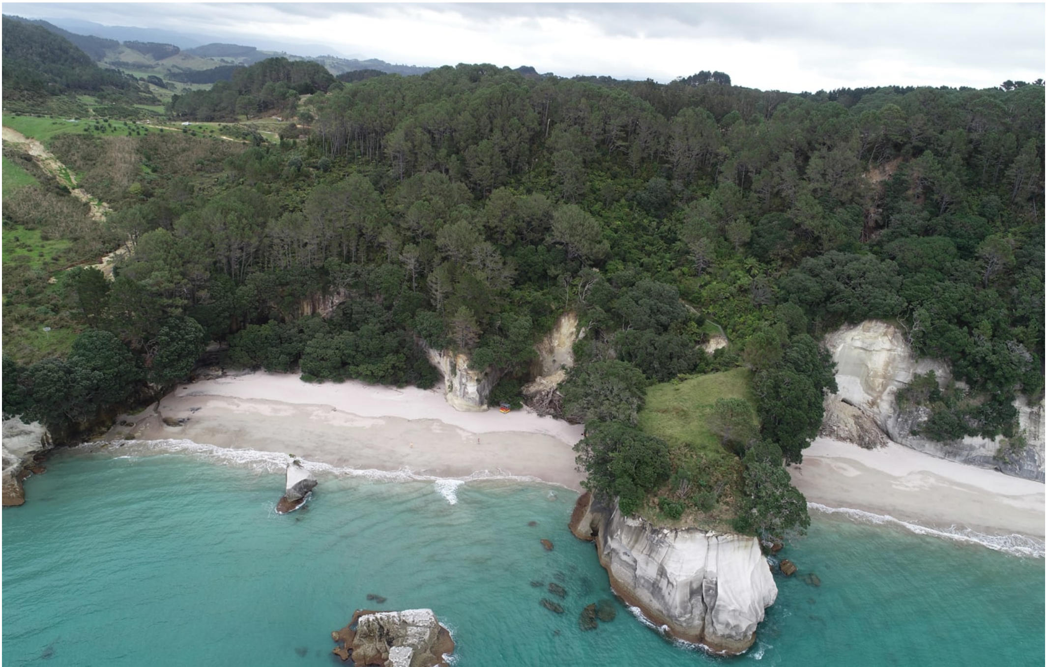
Figure C5 Aerial view of multiple landslides and rockfall at Cathedral Cove Track
