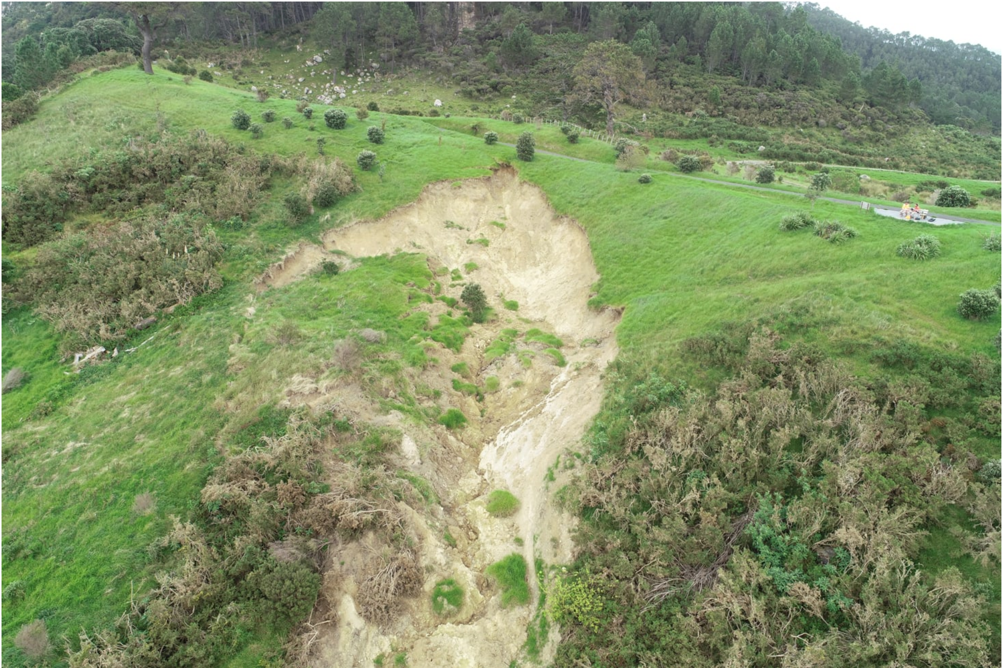
Figure C6 Aerial view of debris flow headscarp. Tension cracks are visible in grass above headscarp (directly below track).
