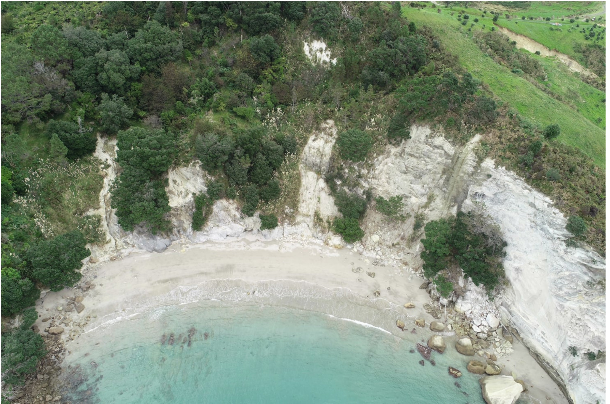
Figure C7 Aerial view of landslides at Stingray Bay
