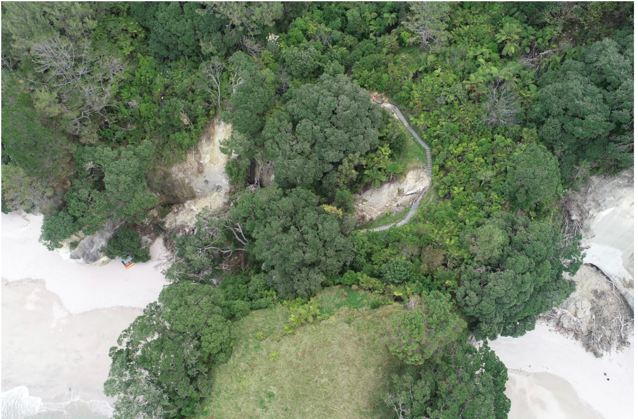
Figure C4 Aerial view of the damage to Cathedral Cove Track
