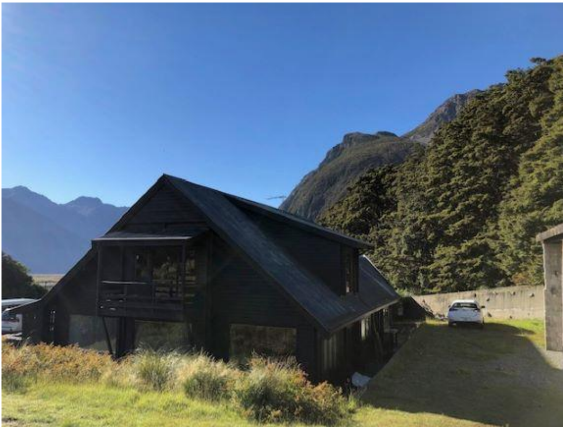
Photo 2 – back view of AGL building
