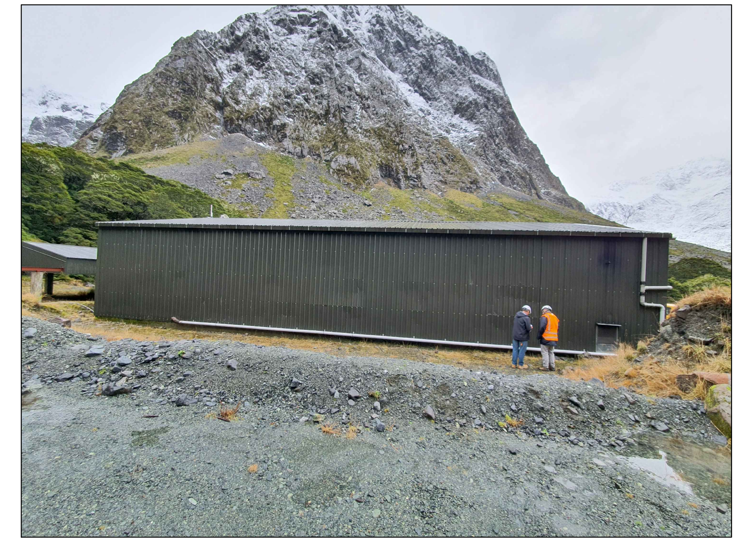
PROPOSED GENERATOR BUILDING LOCATION
