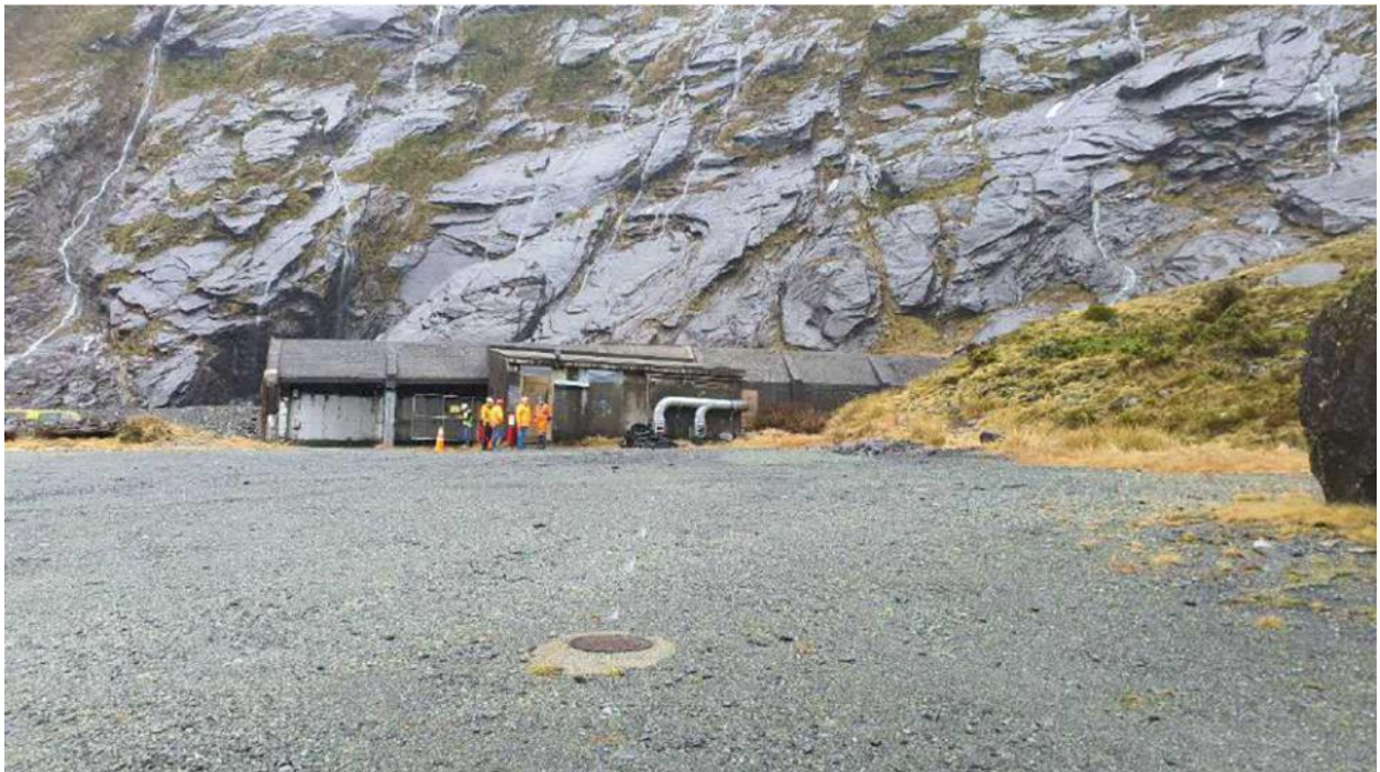
Figure 3: Existing plant room, avalanche shelter and talus slope viewed from car park
