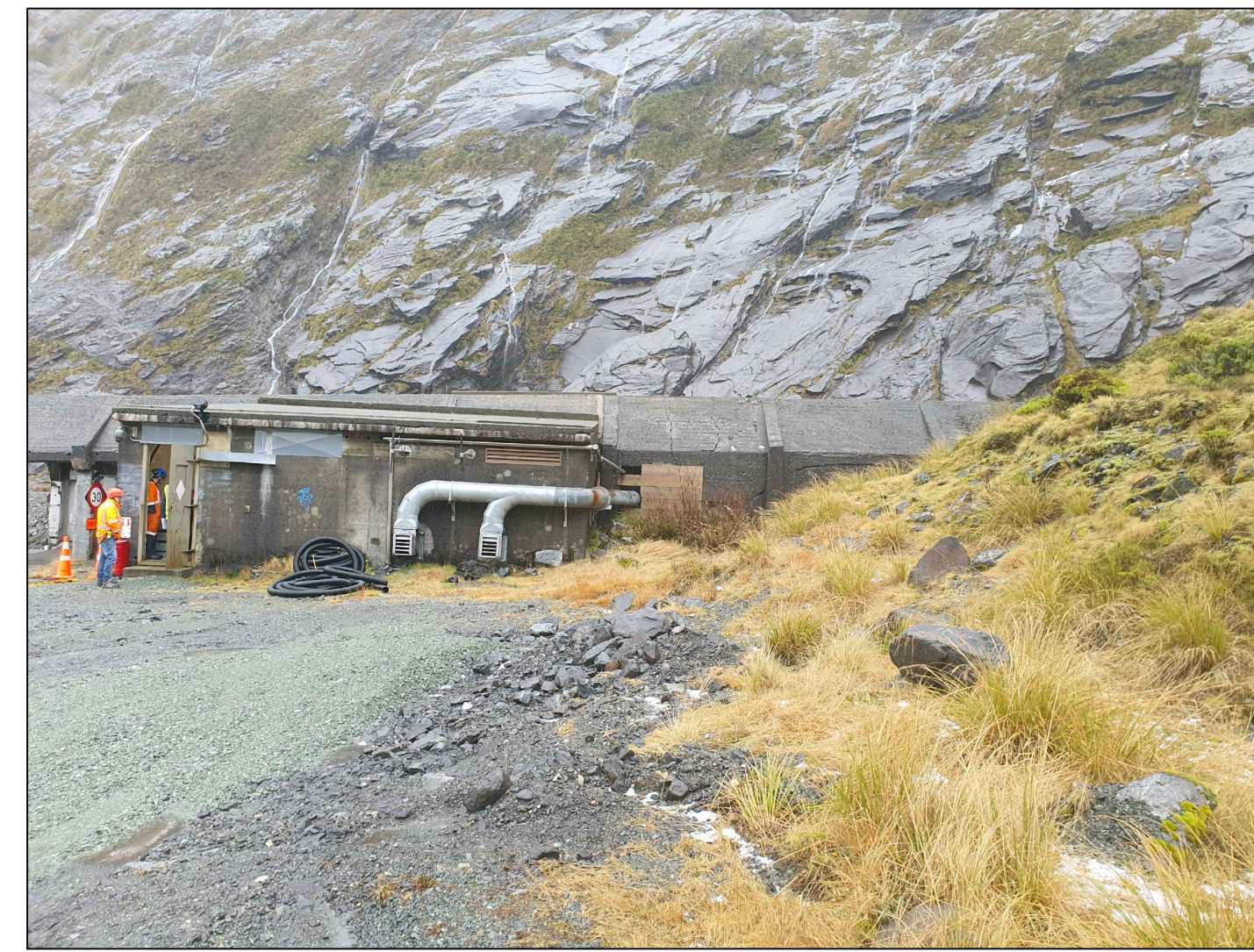
EXISTING AVALANCHE SHELTER AND GENERATOR ROOM
