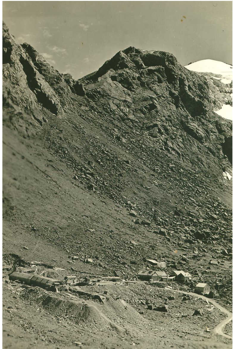
Figure 3-1: Homer Tunnel Construction Work Site, 1937. Source: Downer.
