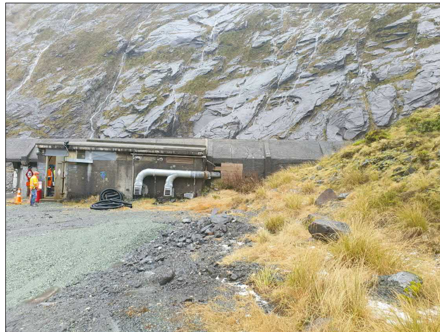
EXISTING AVALANCHE SHELTER AND GENERATOR ROOM
