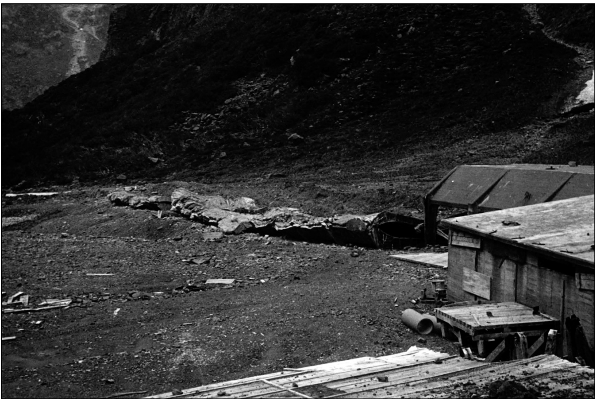
Figure 3. View of collapsed eastern portal avalanche protection, 14 January 1946. 28
