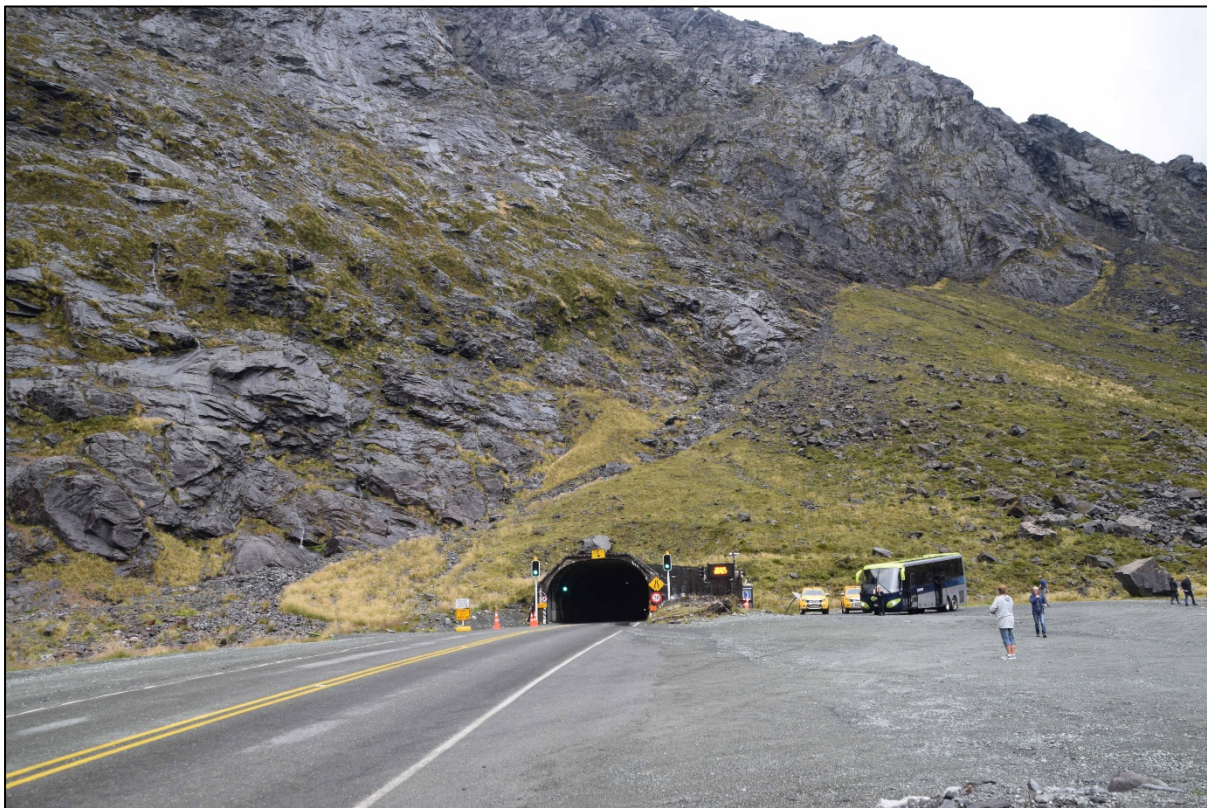
Figure 1. Eastern portal and avalanche shelter, with the concrete plant room visible to the right of the tunnel entrance.
