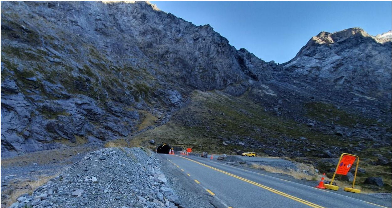
Figure 2: Approaching the eastern portal and avalanche shelter, with the concrete plant room just visible to the right of the tunnel entrance. There are earth bunds either side of the carriageway; that on the left side provides rockfall protection and the one on the right side prevents access to the now-closed car park
