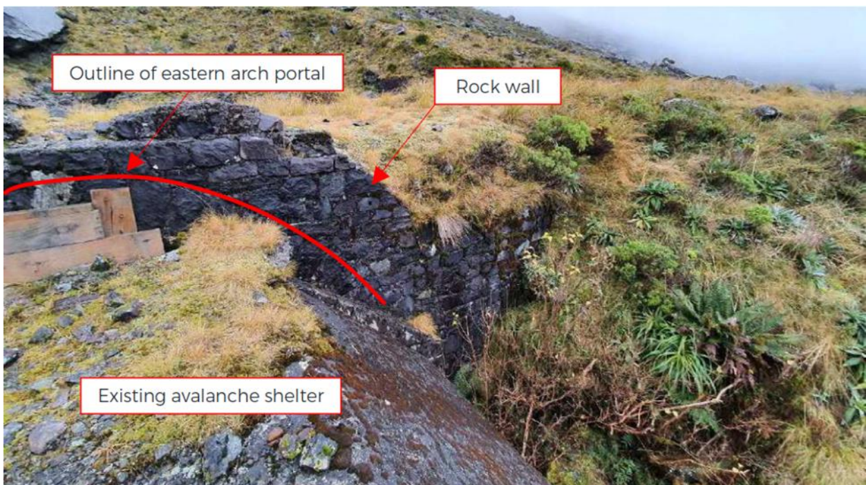
Figure 5: Rock wall at tunnel portal
