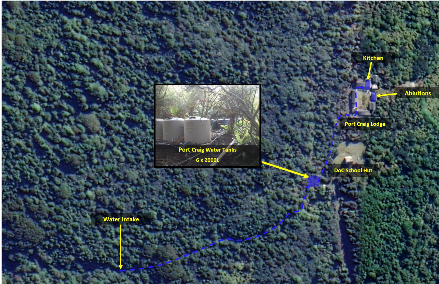
Figure 10 Port Craig water infrastructure
