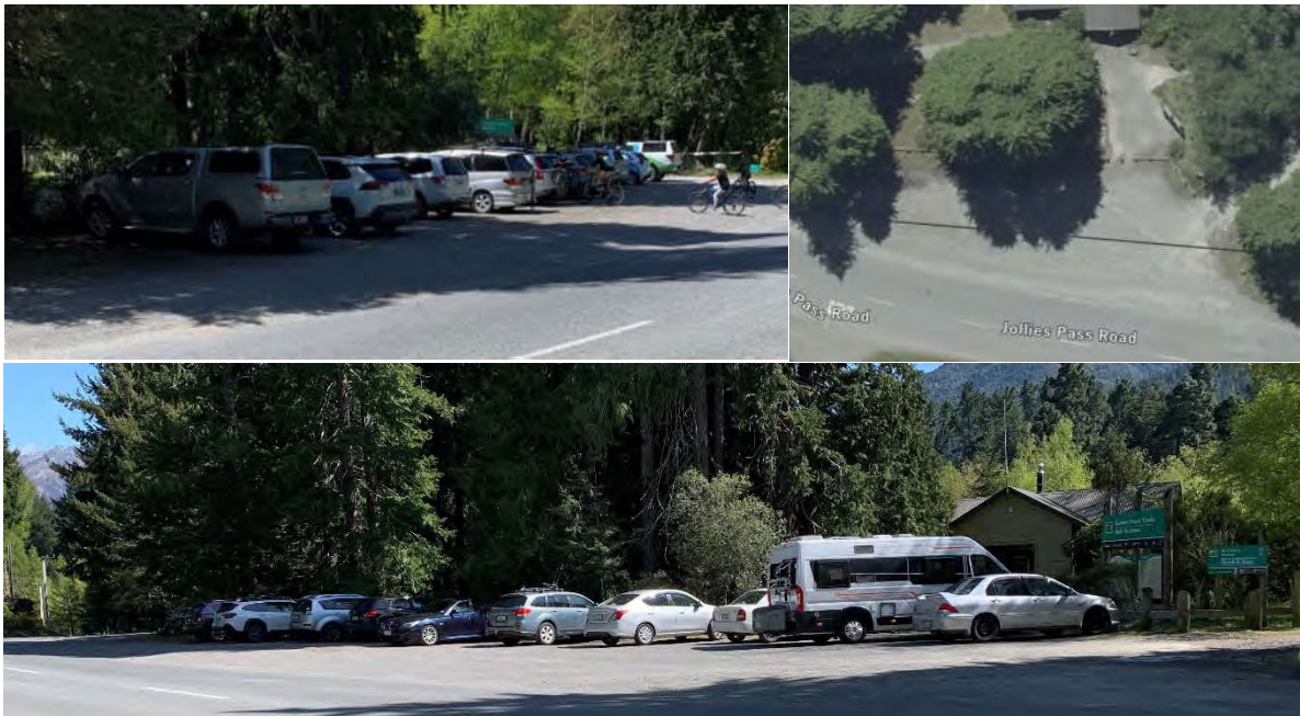
Photograph 5: Area 5 Parking (Top Left: View from West; Top Right: Aerial; Bottom: View from East)
