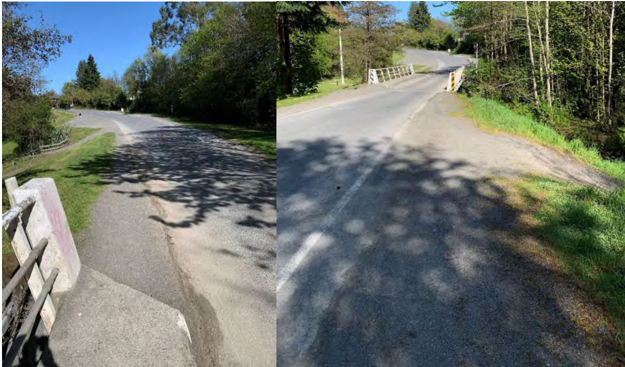
Photograph 8: View of Informal Pedestrian Path on Along Jollies Pass Road (Left: View West Towards Car Park 7; Right: View West Towards Bridge and Pedestrian Footpath on South Side of Bridge)
