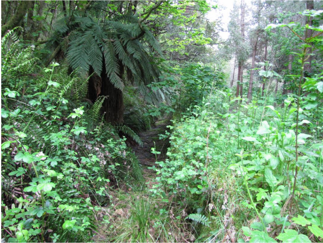
Photo 2: Overgrown Section of Water Race
