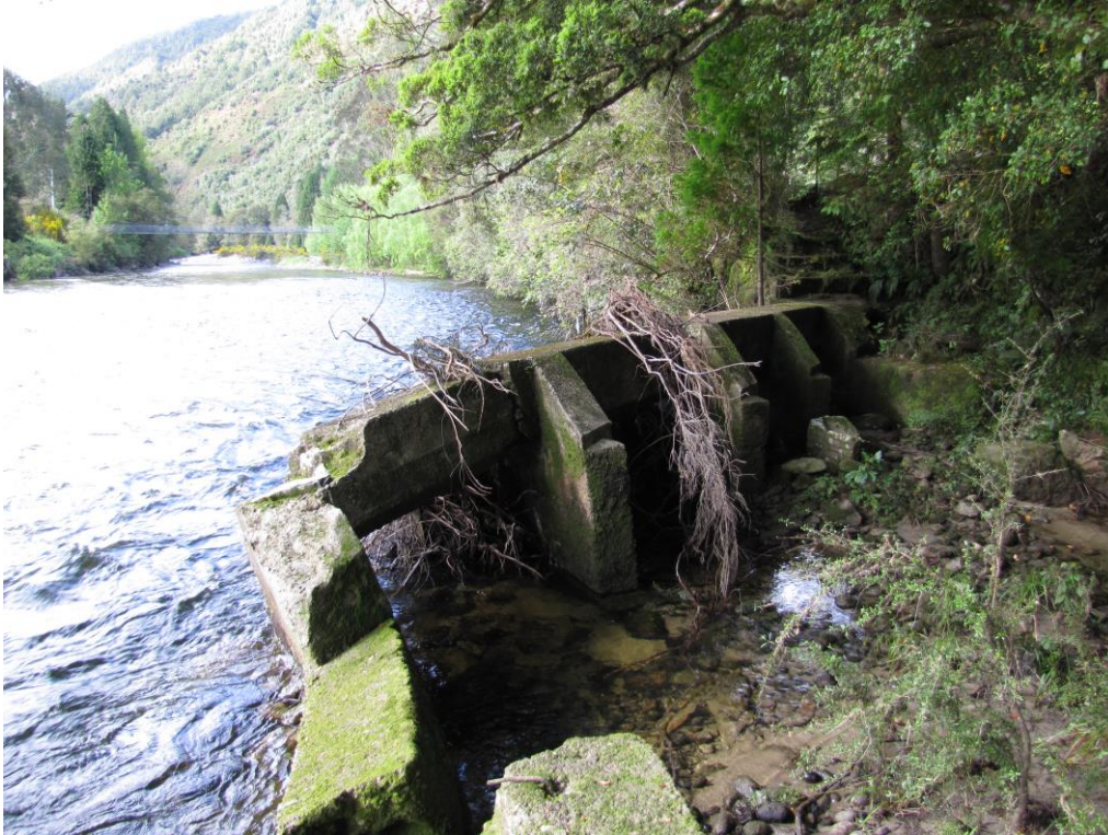
Photo 4: Intake Structure with the Blackspoint Swingbridge in the Background
