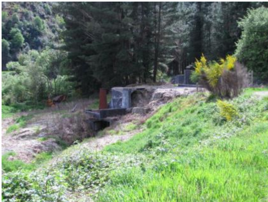
Figure 16. The power house. Image: R. Inwood.
