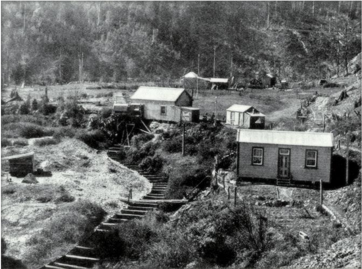
Figure 9. The tail race (foreground), power house (centre) and manager's house (right), 1888. Image supplied by R. Inwood.
