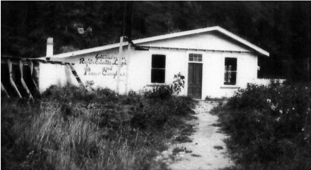
Figure 7. The 1906 power house, looking north.
