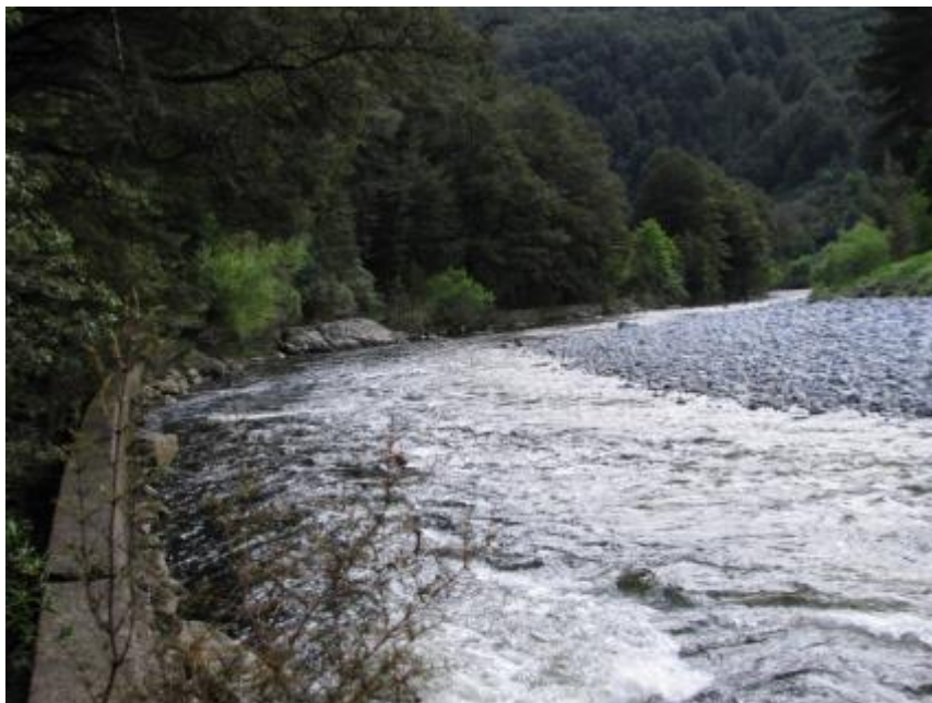
Figure 12. The concrete channel. Image: R. Inwood.
