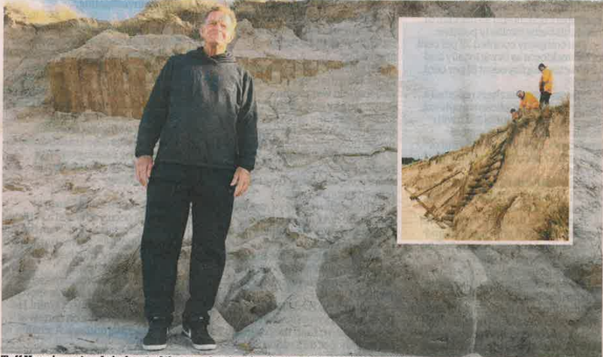
Taff Kennice stands in front of the wooden facing installed in the 1920s at Whangamata Beach Inlet, Beach
