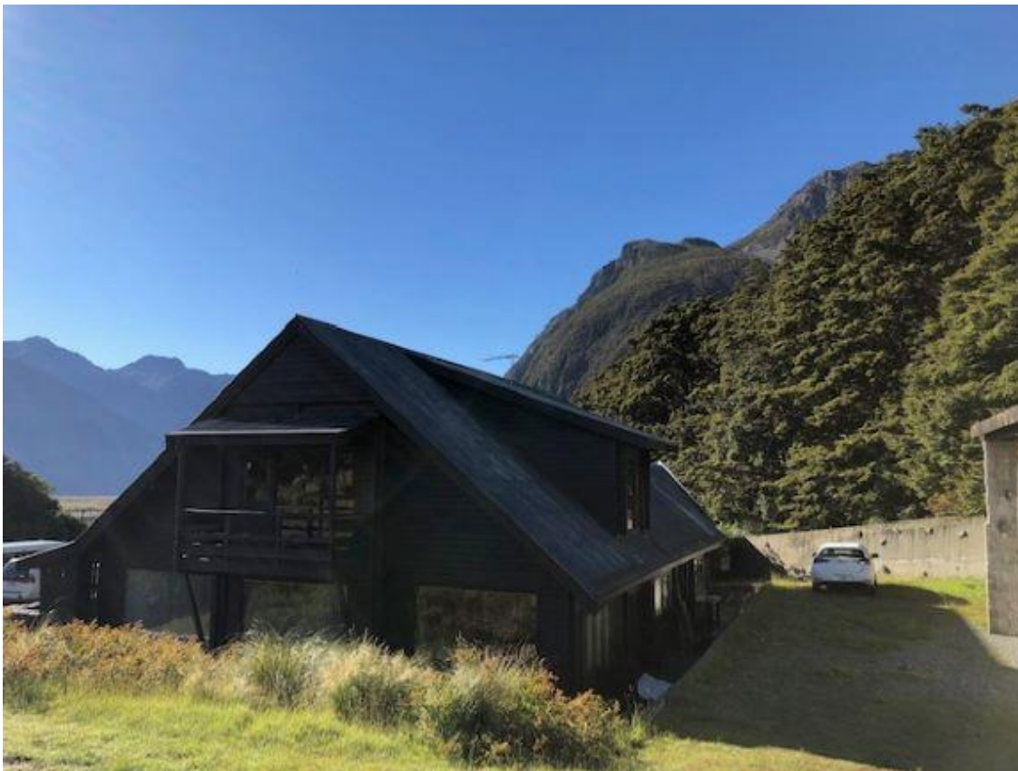
Photo 2 – back view of AGL building
