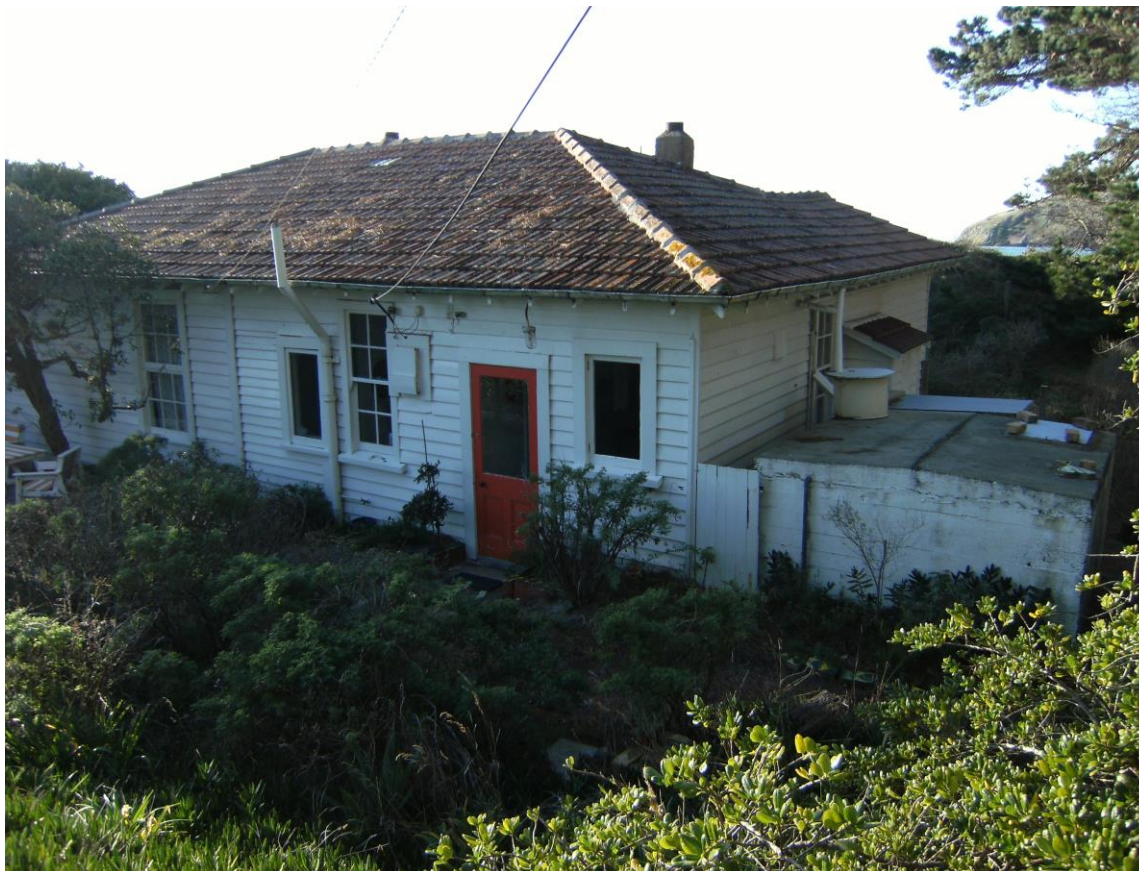
Figure 1: Cottage/pilot house No.3 (July 2015)
